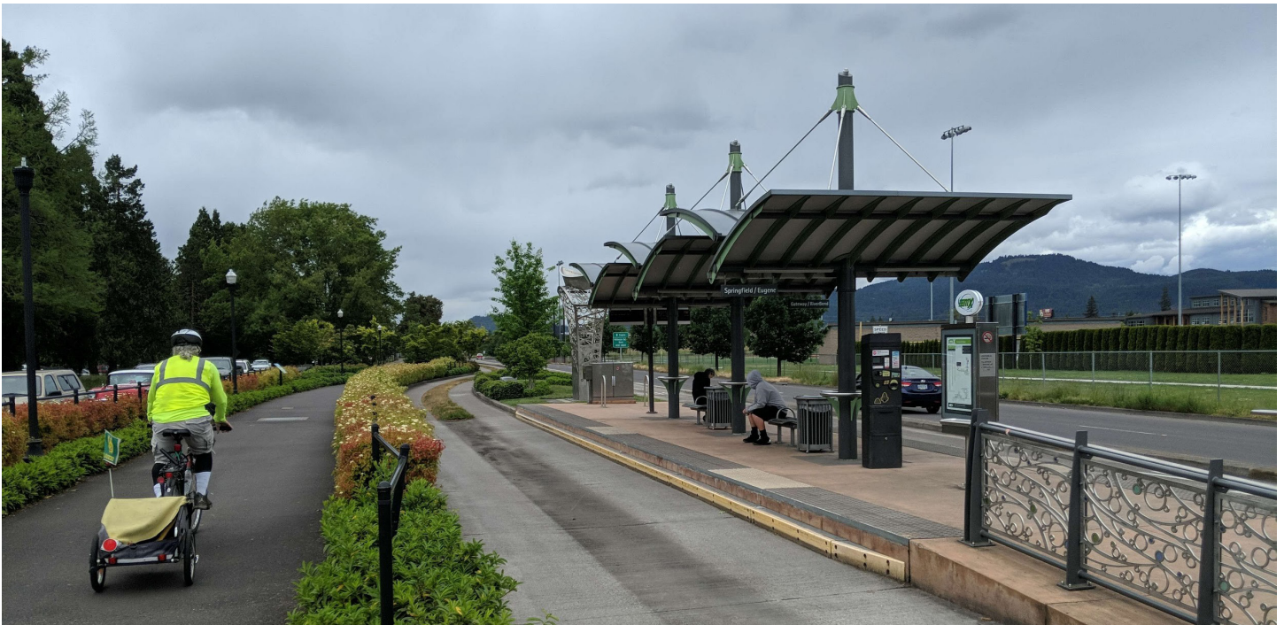
FIG NUM. 25 Centennial Station looking north
