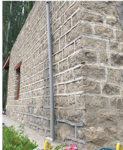
d) Hybrid exposed stone wall: Ashlar masonry wall bonded with mud mortar.
