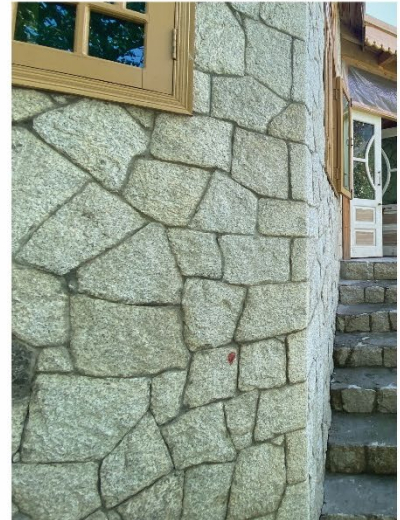
e) and f) Contemporary exposed stone walls: Polygonal masonry walls built with hand-chiseled stones fitted together tightly and bonded with cement mortar.
