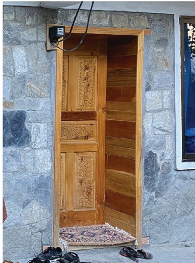
e) and f) Contemporary exposed stone walls: Polygonal masonry walls built with hand-chiseled stones fitted together tightly and bonded with cement mortar.
