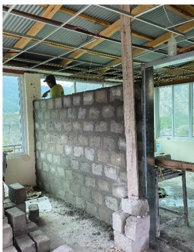
h) Contemporary CMU wall with metal sheet roof: Under construction metal sheet roof and CMU wall.
