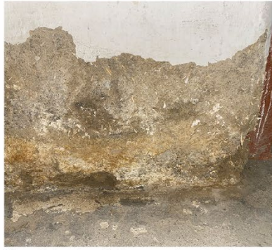
b) Traditional wall: Close-up of mud and straw plaster revealed beneath chipped white paint.
