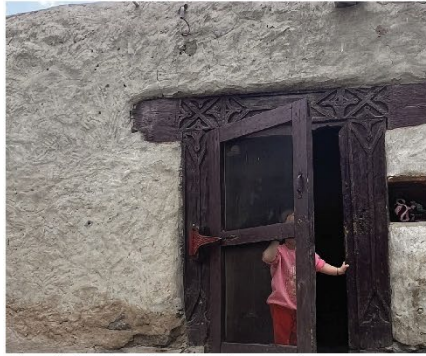
a) Traditional wall: Mud and straw plaster on a traditional wall.
