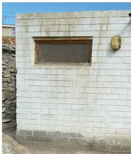
g) Contemporary CMU wall: Wall built with CMU and plastered with cement-sand plaster on both interior and exterior.
