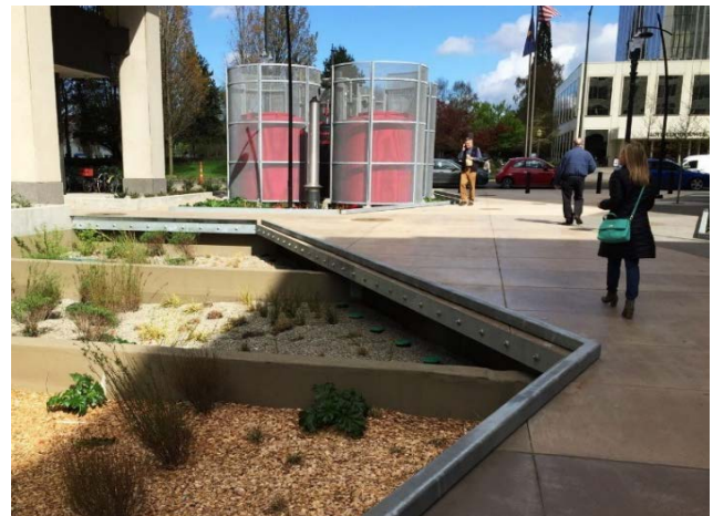
Figure 5: Hassalo on 8 th , constructed wetlands
