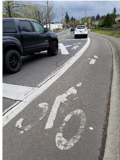
Figure 7: There is no buffer between cars and bicycles on Hall Boulevard
