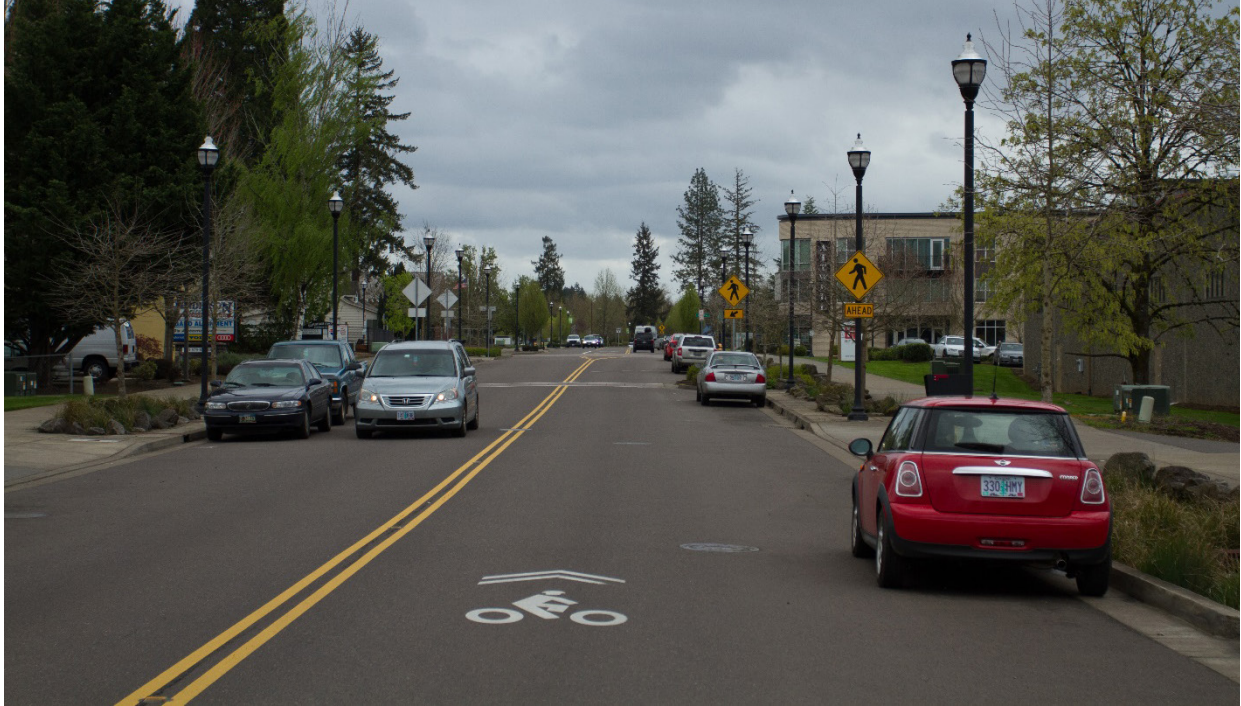
Figure 11: POINT F. Burnham Street looking south. Shared roadway with some bike markings on the pavement (Photo credit: Ethan Zagorec-Marks)
