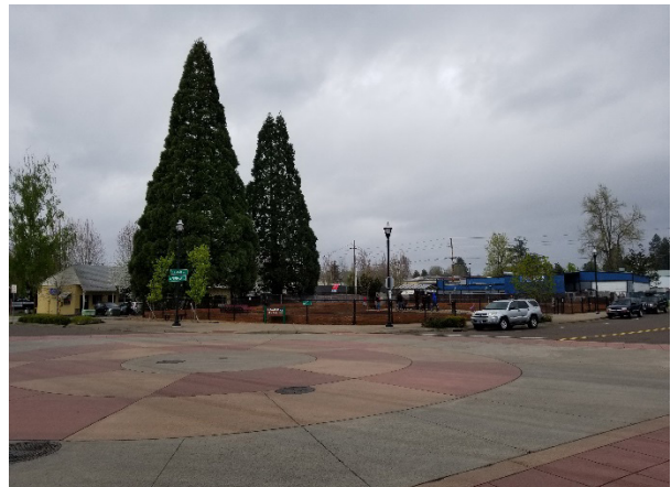
Figure 3: The intersection of Burnham Street and Ash Avenue changes pavement pattern and material to emphasize pedestrian crossing
