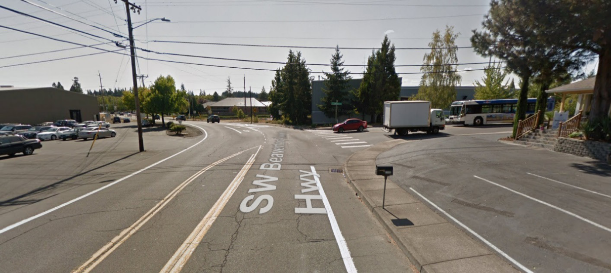
Figure 7: POINT C. Hall Boulevard and Commercial Street intersection looking west. Large intersection with no continuous bike lane markings (Photo credit: Google)
