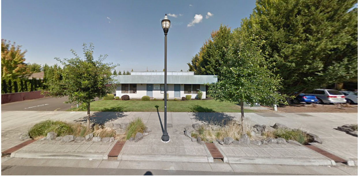
Figure 2: An example of Tigard's new stormwater infrastructure
