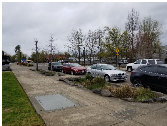
Figure 10: Bioswales as buffer zone along Burnham
