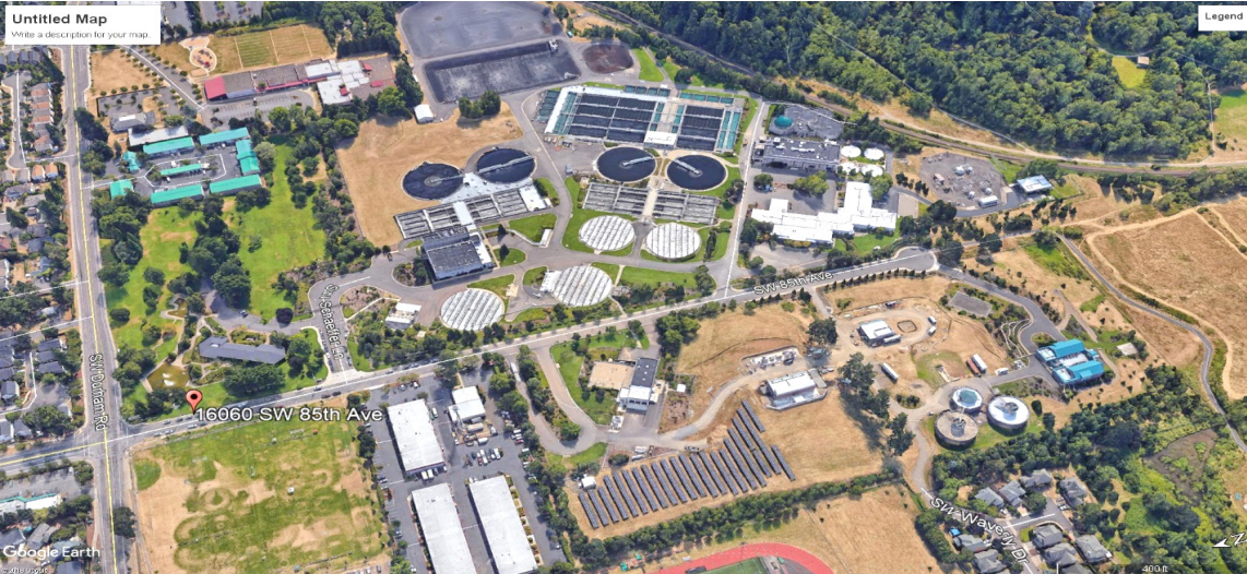
Figure 6: Durham Treatment Plant – serving Beaverton, Durham, King City, Sherwood, Tigard, and Tualatin (image from Google Earth Pro™)
