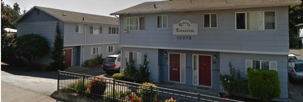
Figure 6: Townhouses along SW Hall Boulevard
