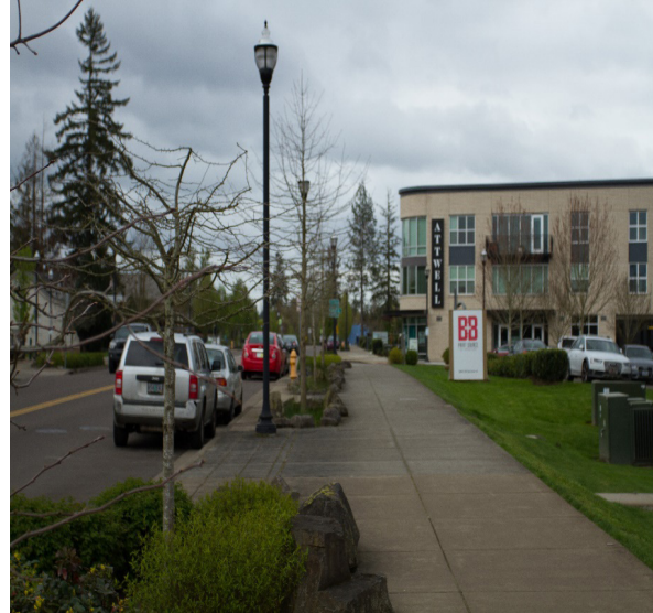
Figure 3: Burnham Street, a recently developed street in Tigard. Photo by Ethan Zagorec-Marks
