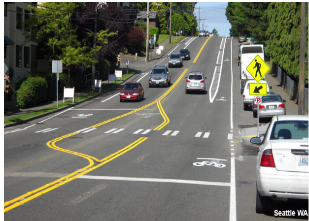
Figure 2: Buffered bike lane in Seattle, WA (Photo credit: NACTO)
