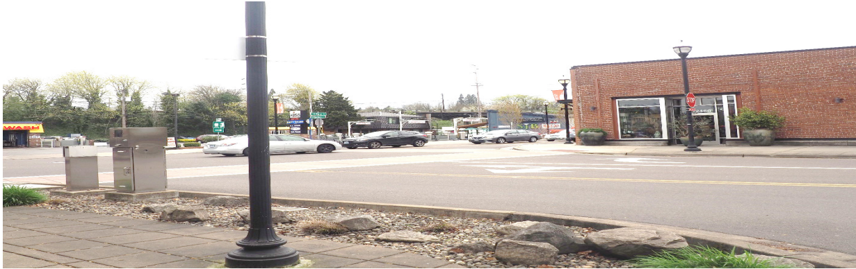
Figure 3: Passive drainage systems (photo by Nate Carden)
