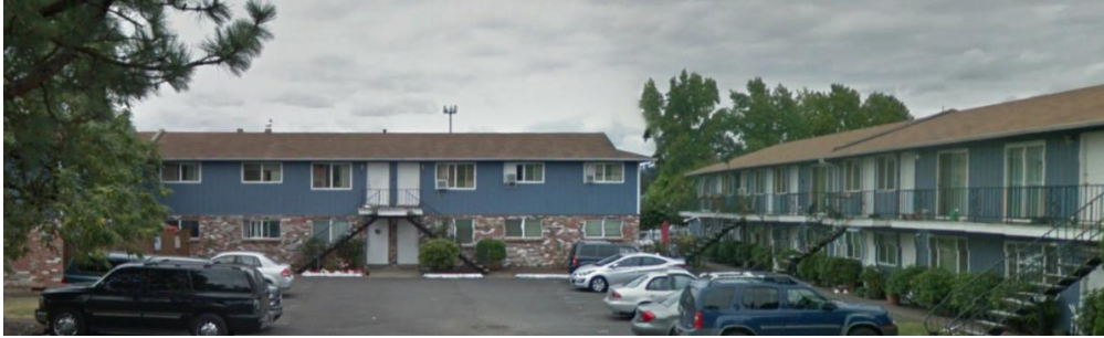
Figure 5: Two story stacked duplexes along Scoffins Street
