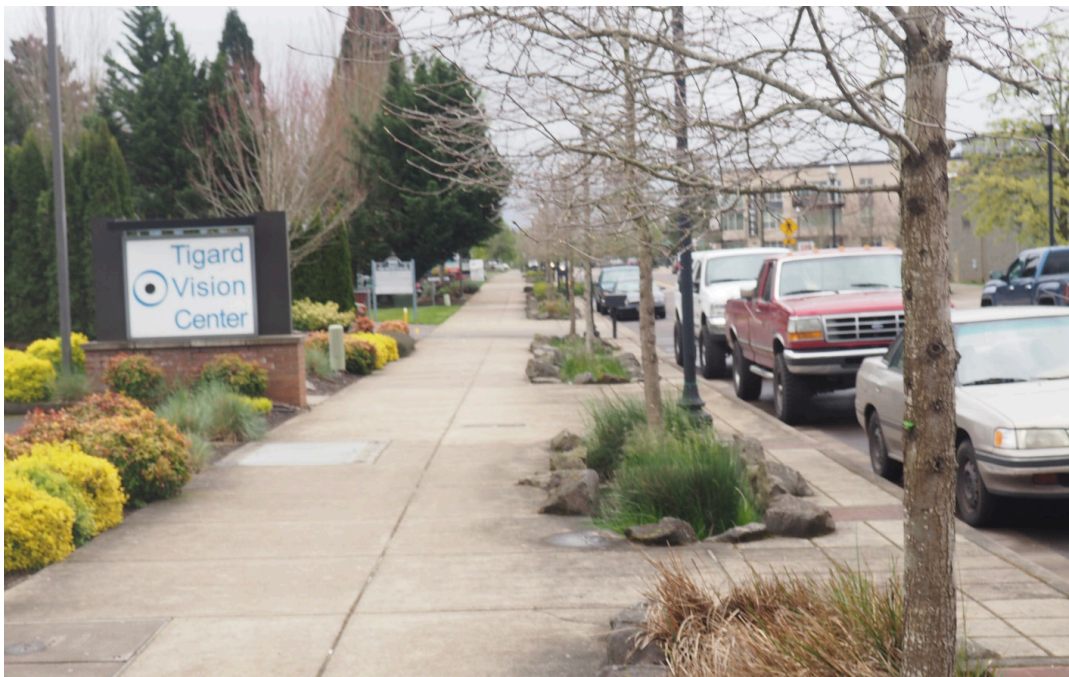
Figure 4: Stormwater planters (photo by Nate Carden)
