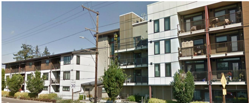
Figure 7: The Knoll at Tigard apartment building
