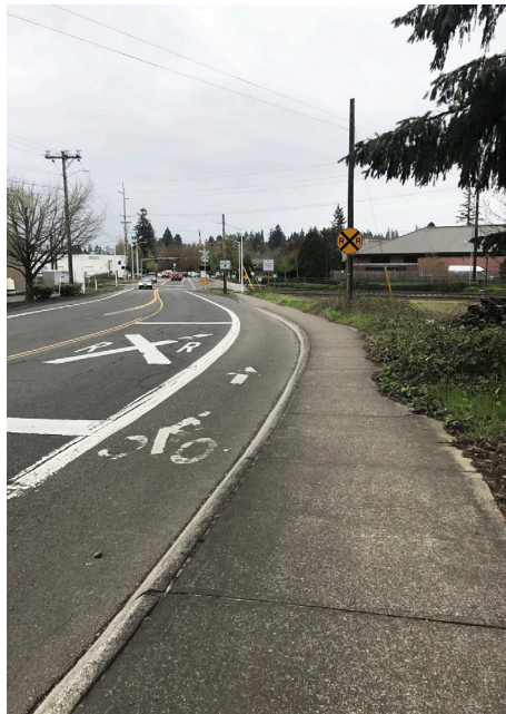
Figure 3: Looking southwest down SW Hall Boulevard
