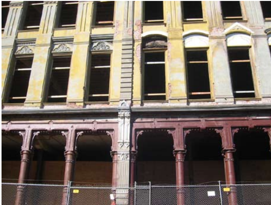
The renovation of this building façade maintains the building walls in place while the windows have been removed for repair.
