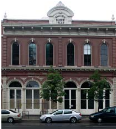
The Smith Block and Bickel Block are examples of appropriate alterations and renovations which repaired rather than replaced most of the original materials.
