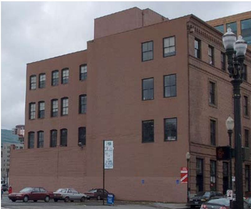
This building on SW First Avenue demonstrates how in an appropriate alteration the majority of the wall area is preserved and when new windows are introduced they are simpler than the original windows.
