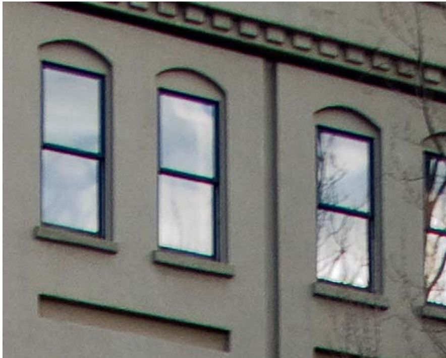
New buildings should employ window spacing and styling similar to this historic building.
