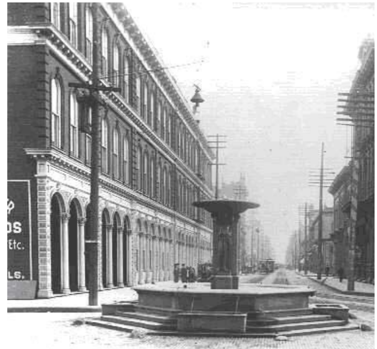
This building at SW Ash and First was constructed over a period of time through a number of additions, although it was designed to appear as a single multi-module building.
