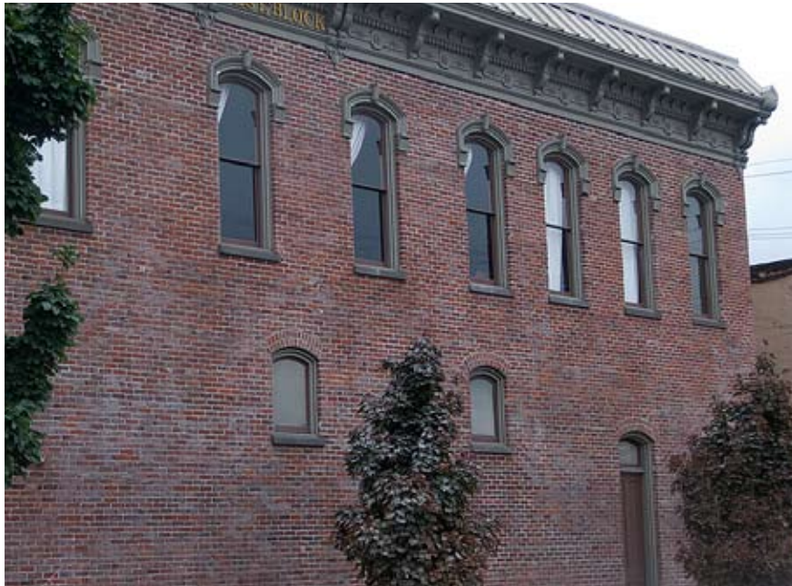
The renovation of the West's Block required the removal, repair, and reinstallation of all of the upper story windows.
