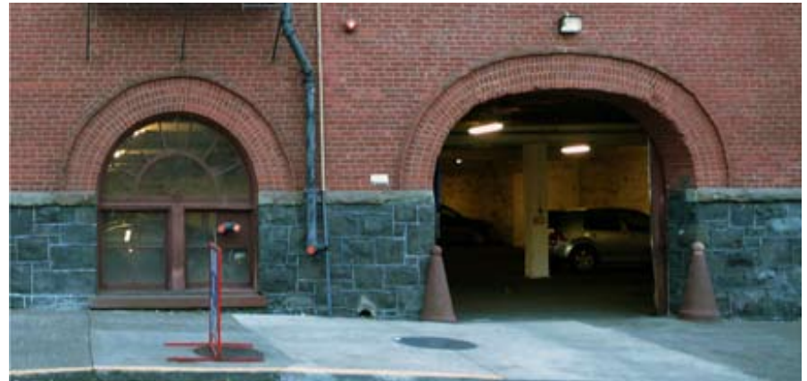
This garage entry on NW 11th Avenue is an example of a garage entry using the same design vocabulary used for the rest of the building.
