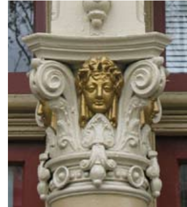
30 NW 1st, Blagen Block. Cast Iron Column Capital
