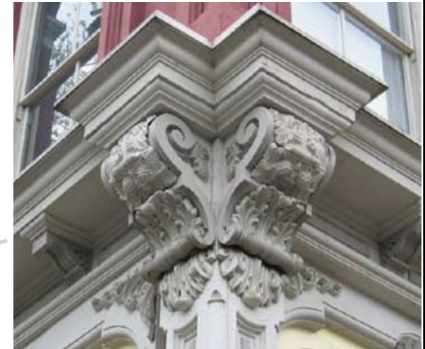
In this example, missing cast iron pieces were fabricated from contemporary materials and installed to complete the building detailing
