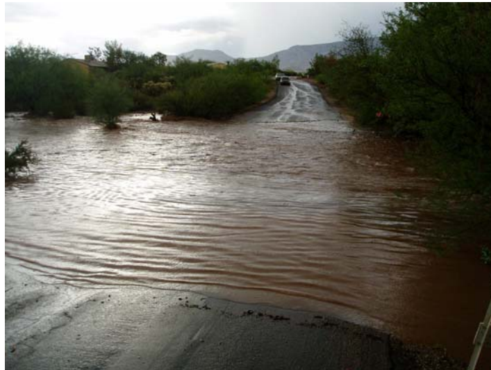
Photo 2.1. July 24, 2007, street flooding
