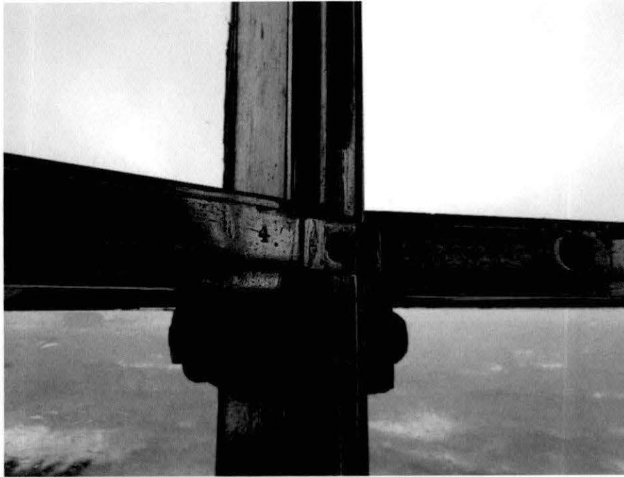
Figure 4-11: Cape Meares Lantern mullions individually numbered for assembly (Photo by Author)
