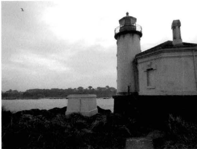
Figure 4-6: Image showing the steep stairway entrance into the Coquille River lighthouse (Photo by Author)
