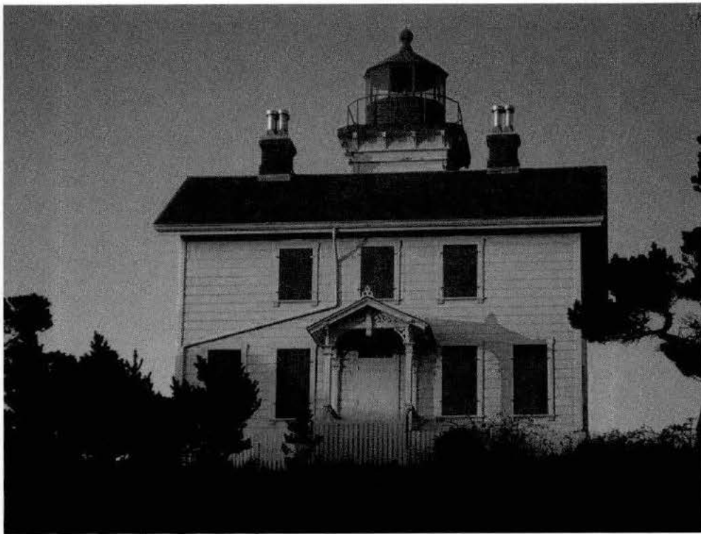
Figure 2-4: Yaquina Bay Lighthouse, Newport, 2010 (Wikimedia Commons)
