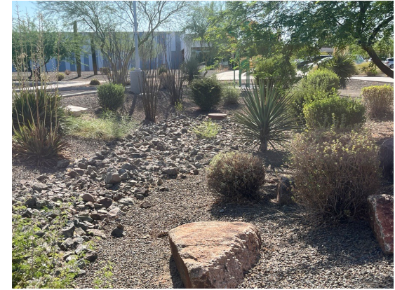
This shallow channel directs, slows, and helps filter stormwater runoff. It also contributes to habitat. Source: City of Tempe, AZ.
