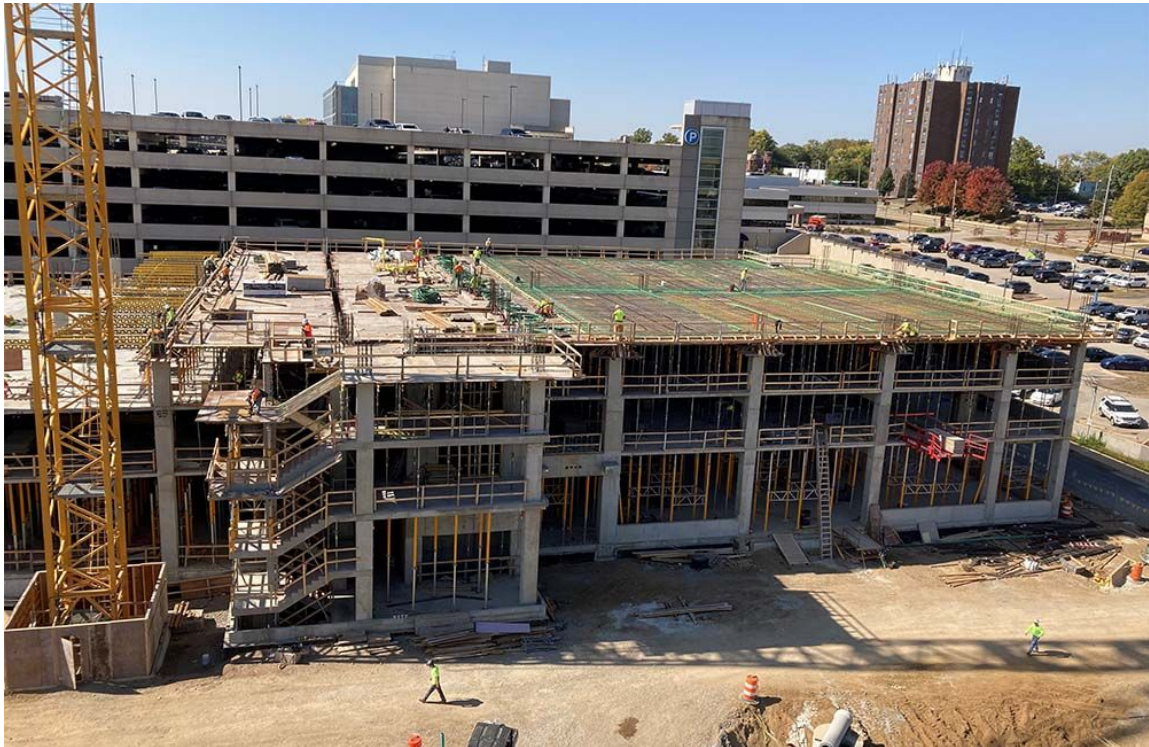
IMAGE 8: CONCRETE COMMERCIAL CONSTRUCTION 1073
