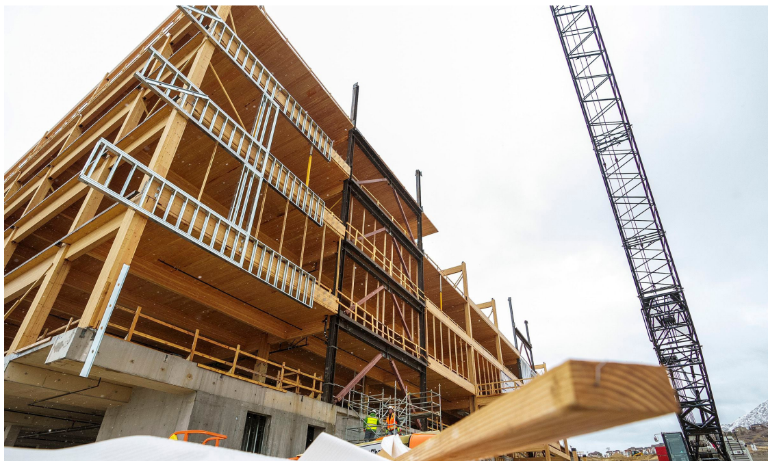
IMAGE 7: CROSS LAMINATED TIMBER OVER COMMERCIAL PLATFORM 1072
