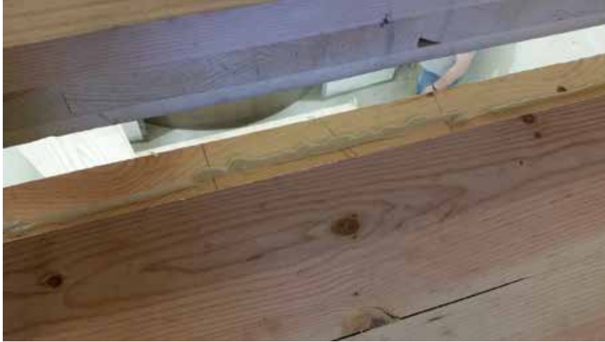
Figure 5 – Adhesive at shiplap joint
