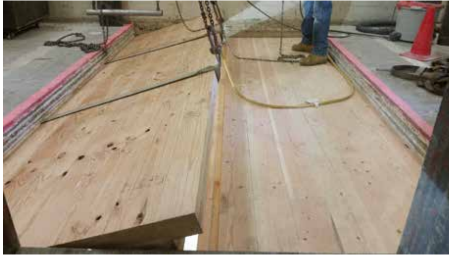
Figure 3 – Installation of cross-laminated timber base slab
