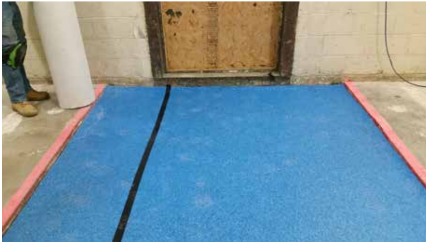
Figure 8 – Carpet pad installed
