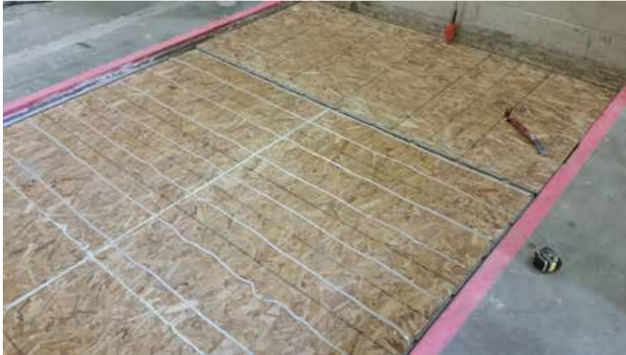
Figure 7 – Oriented strand board layers partially installed
