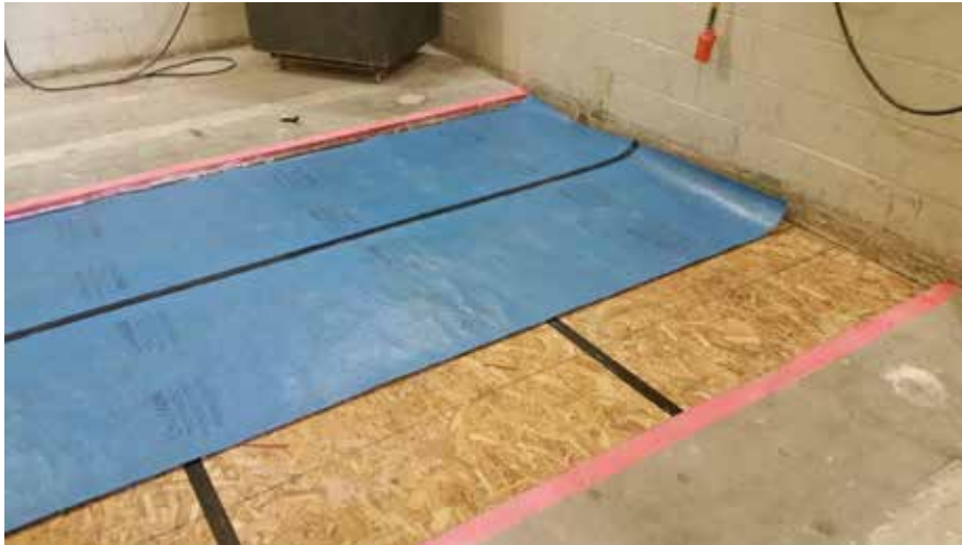
Figure 8 – Recycled cotton underlayment partially installed
