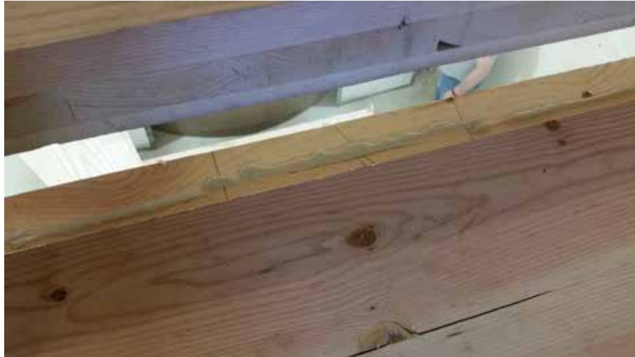
Figure 5 – Adhesive at shiplap joint
