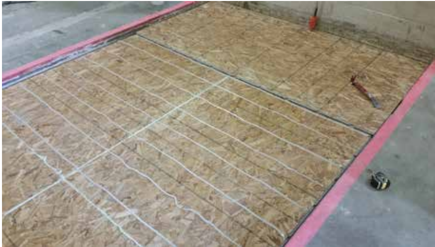
Figure 7 – Oriented strand board layers partially installed
