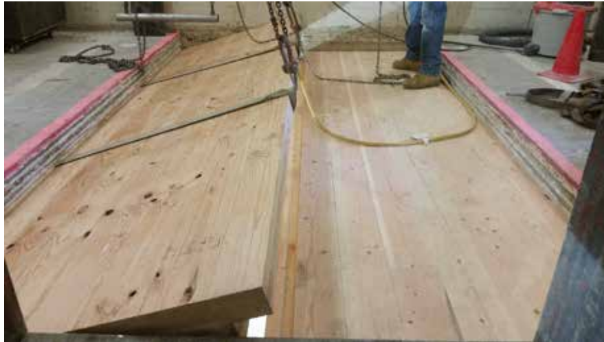
Figure 3 – Installation of cross-laminated timber base slab
