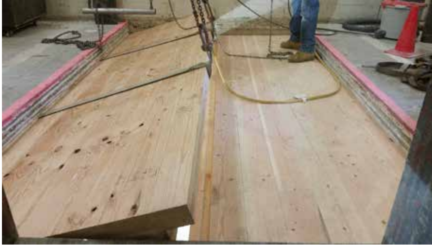
Figure 3 – Installation of cross-laminated timber base slab
