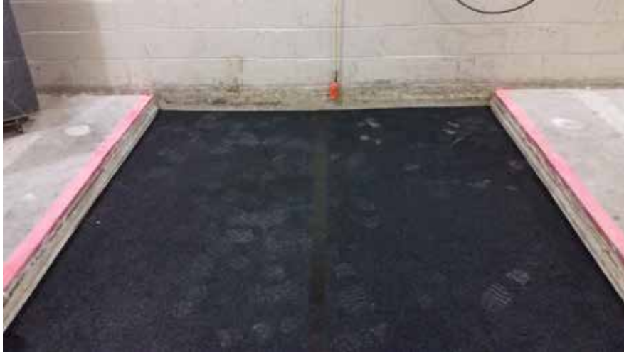
Figure 5– Composite flooring layer 1 installed over base slab
