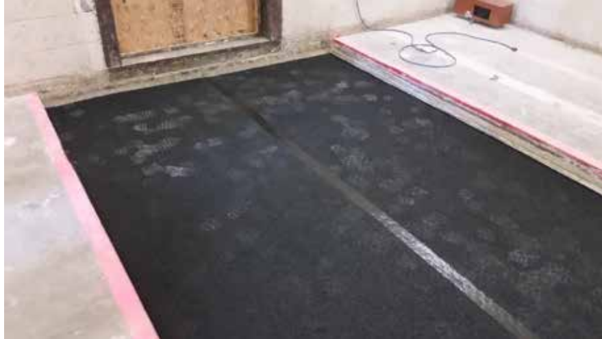
Figure 5 – Composite flooring layer 1 installed
