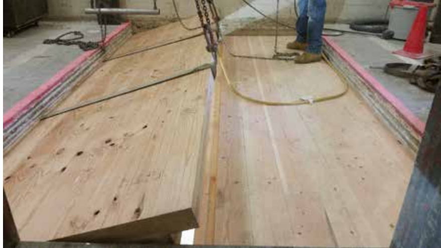
Figure 3 – Installation of cross-laminated timber base slab
