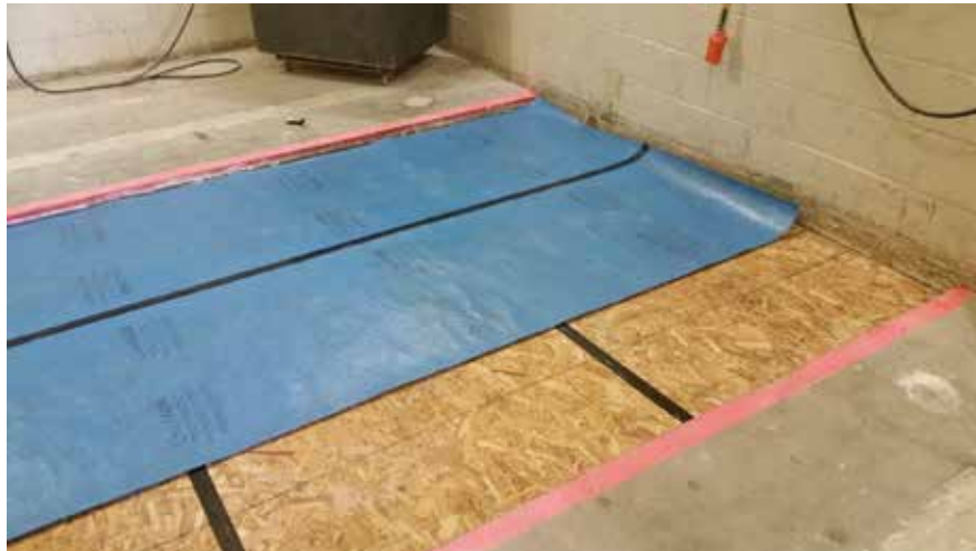
Figure 8 – Recycled cotton underlayment partially installed
