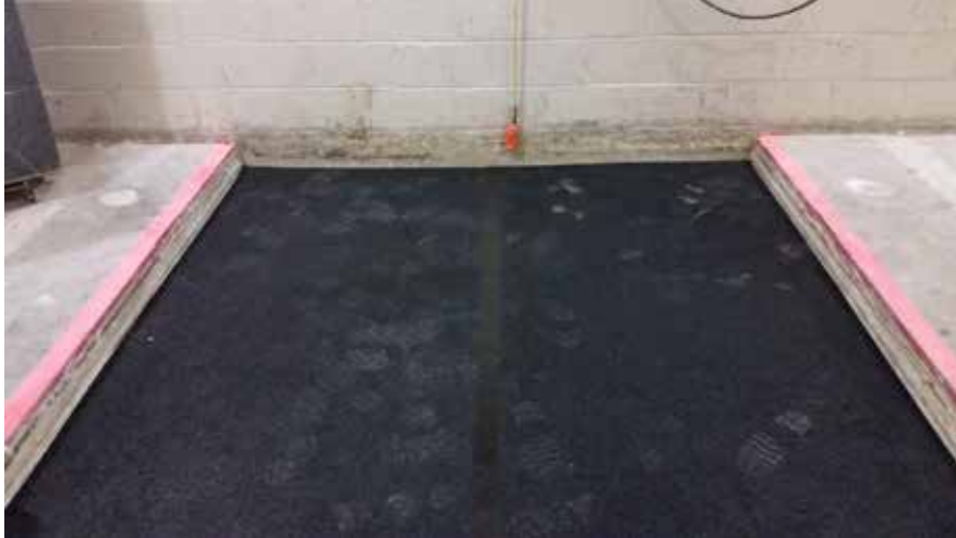
Figure 5– Composite flooring layer 1 installed over base slab
