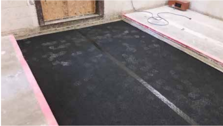
Figure 5 – Composite flooring layer 1 installed
