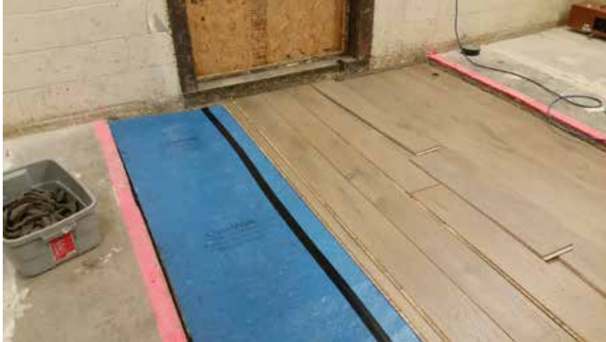
Figure 9 – Engineered wood flooring partially installed
