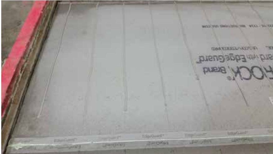
Figure 6 – Typical sealant and adhesive application on cement board layers
