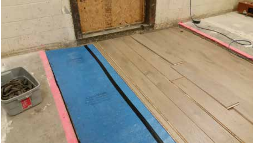
Figure 9 – Engineered wood flooring partially installed
