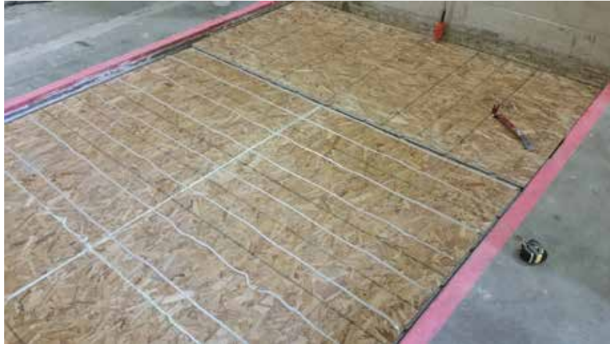
Figure 7 – Oriented strand board layers partially installed
