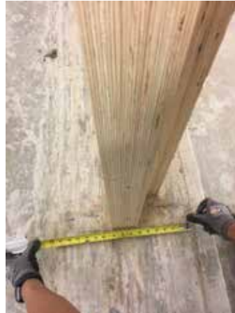
Images this page: the process of receiving the MPP at testing lab, installing and sealing in test opening and assembly build up.
