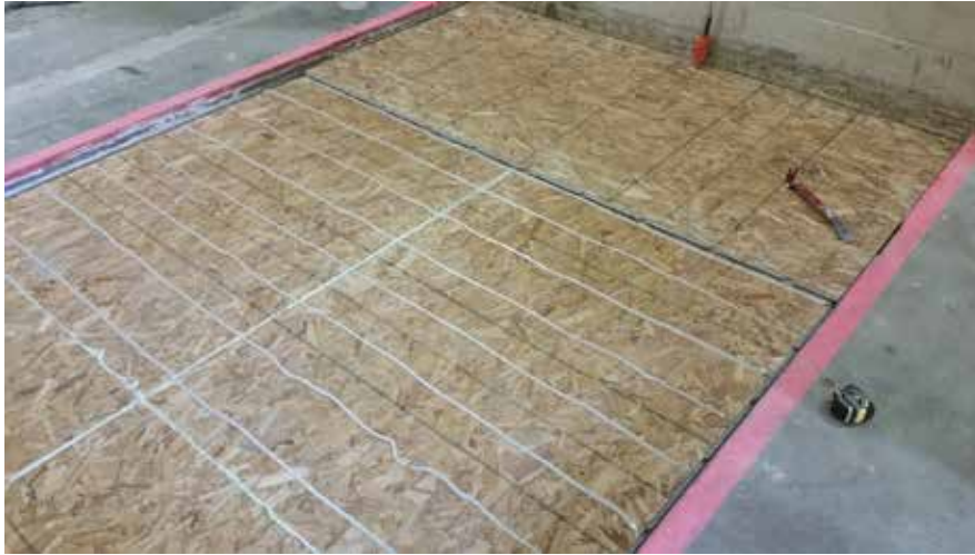
Figure 7 – Oriented strand board layers partially installed
