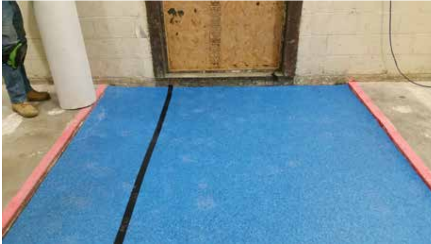
Figure 8 – Carpet pad installed
