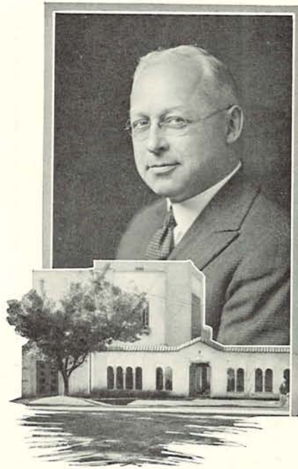
DEAN ELLIS F. LAWRENCE FACADE OF ART BUILDING
