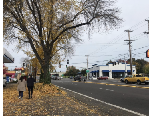
Old Station Site: River Road and Silver Lane Intersect
