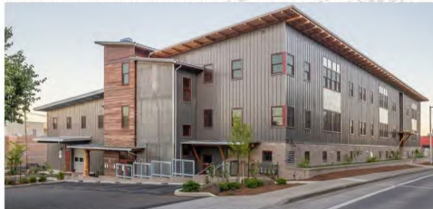
Source: Essex General Construction – Mahonia Building (2019)
