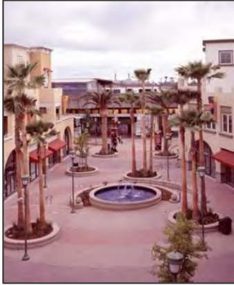
Figure 5.01: Fruitvale Station, completed
