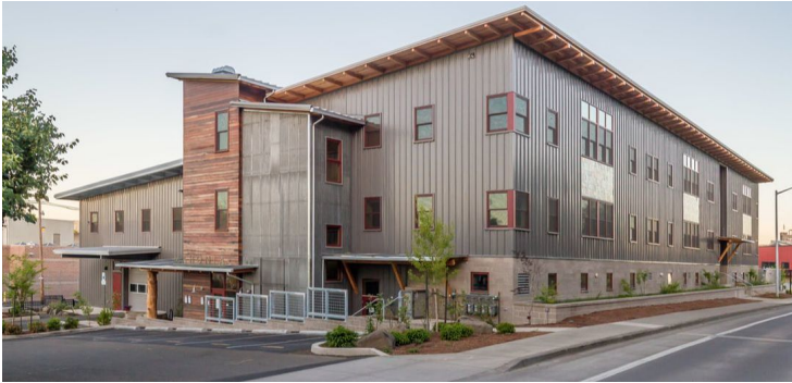
Source: Essex General Construction – Mahonia Building (2019)
