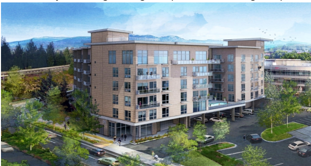
Source: Essex General Construction – 35 Club Road (2019)
