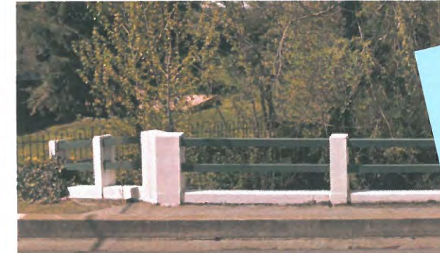
Weston - Existing fence at bridge over stream
