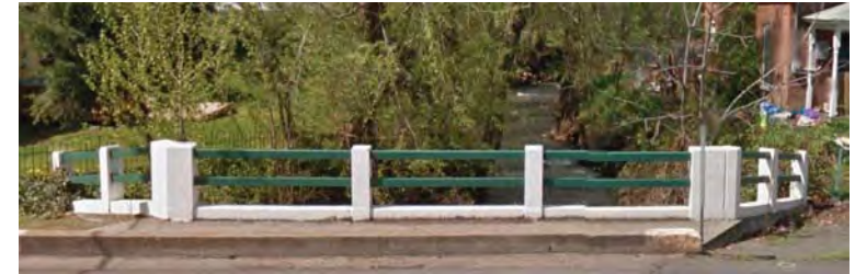
Weston - Existing fence at bridge over stream
