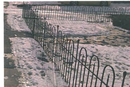
Weston - Existing residential fence
