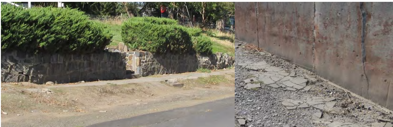
Figure 8 – Retaining Wall Examples (Source: Anderson-Perry & Associates, Inc.)
