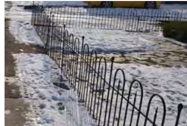
Weston - Existing residential fence
