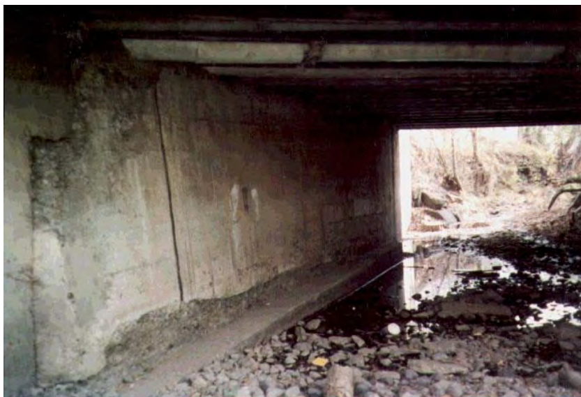
Figure 11 – Underside of Water Street Bridge (Source: Anderson-Perry & Associates, Inc.)
