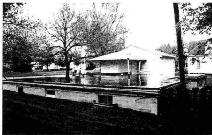
Figure 82. Fee basement house. The relationship of the basement house to the garage and entrance superstructure is a character-defining feature. Photo by author.
