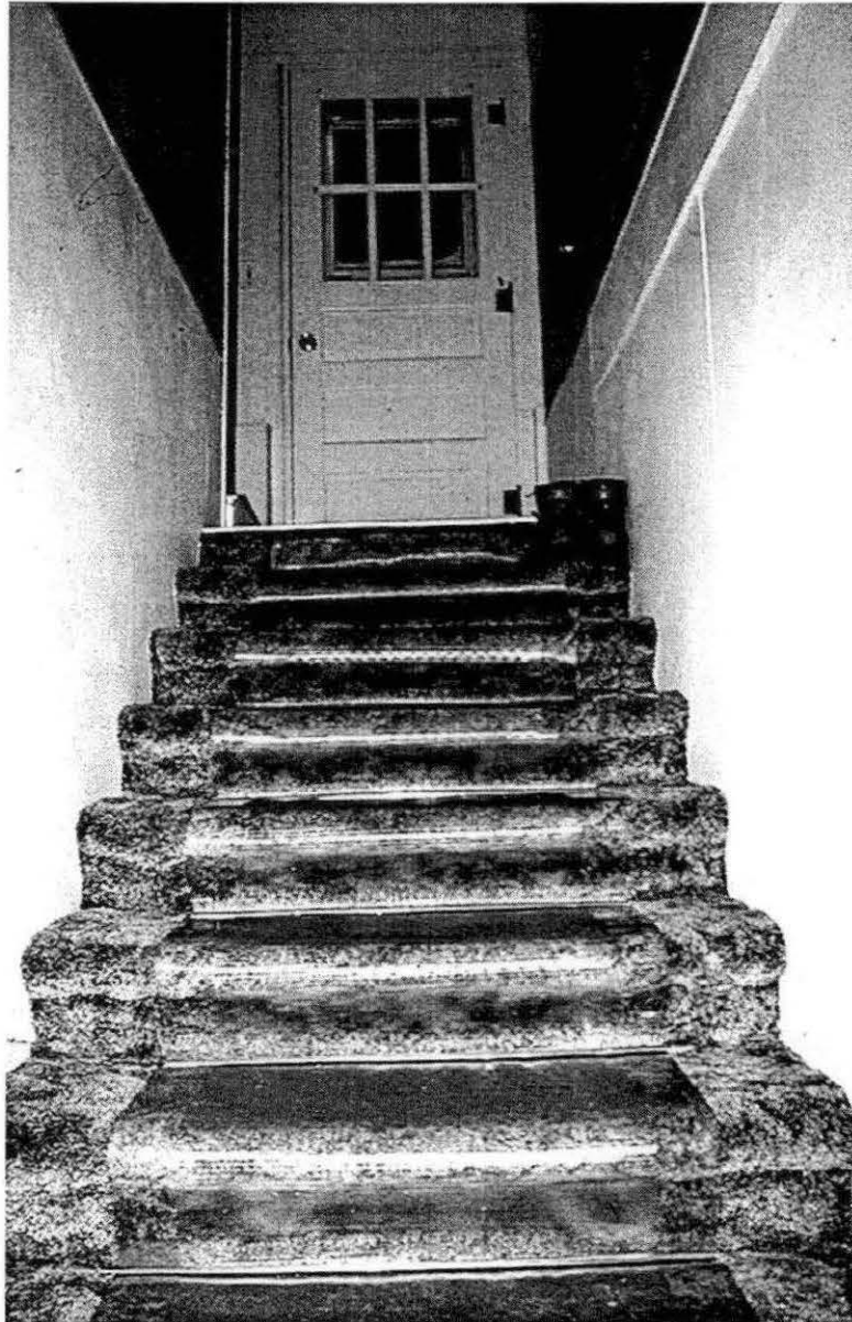
Figure 91. Tokle house original basement entrance stairway. Photo by author.
