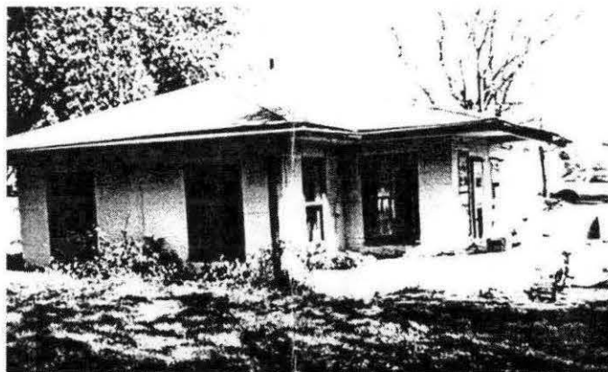
Figure 75. Full-height elevation of basement house at 2200 South Hawthorne, Sioux Falls, South Dakota. Photo courtesy of Sioux Falls Community Development office
