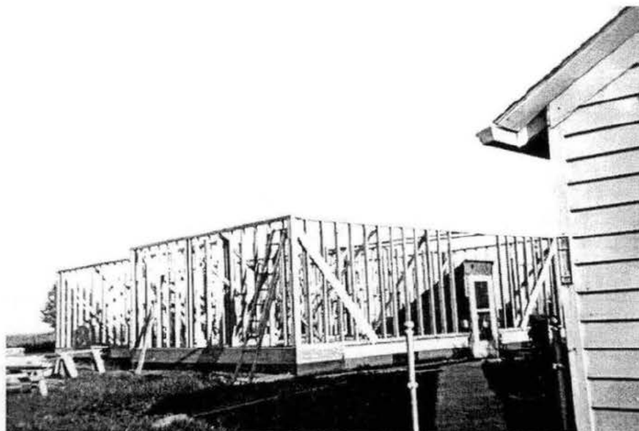
Figure 41. Rikansrud house superstructure under construction, 1954. Note shed entrance to basement house, partially obscured by framing. Photo courtesy of Olive Rikansrud.
