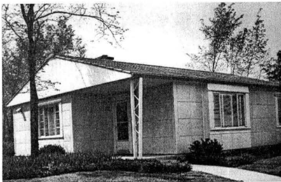
Figure 12. A Lustron house. Source: H. Ward Jandl, Yesterday's Houses of Tomorrow (Washington, DC: The Preservation Press, 1991), 184.
