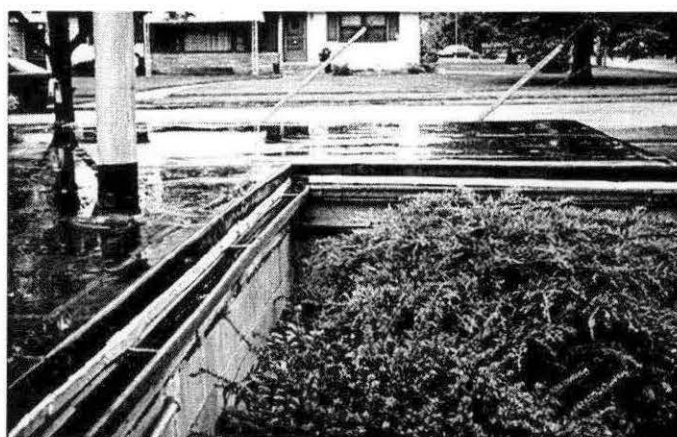
Figure 83. Flat roof of Fee basement house. Photo by author.
