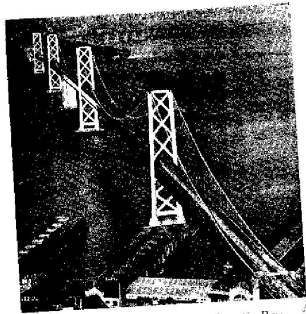
IN SAN FRANCISCO, the gigantic Bay span, world's largest (shown above), and the Golden Gate Bridge, nearing completion, now number among the thrilling sights of this well-loved city.
