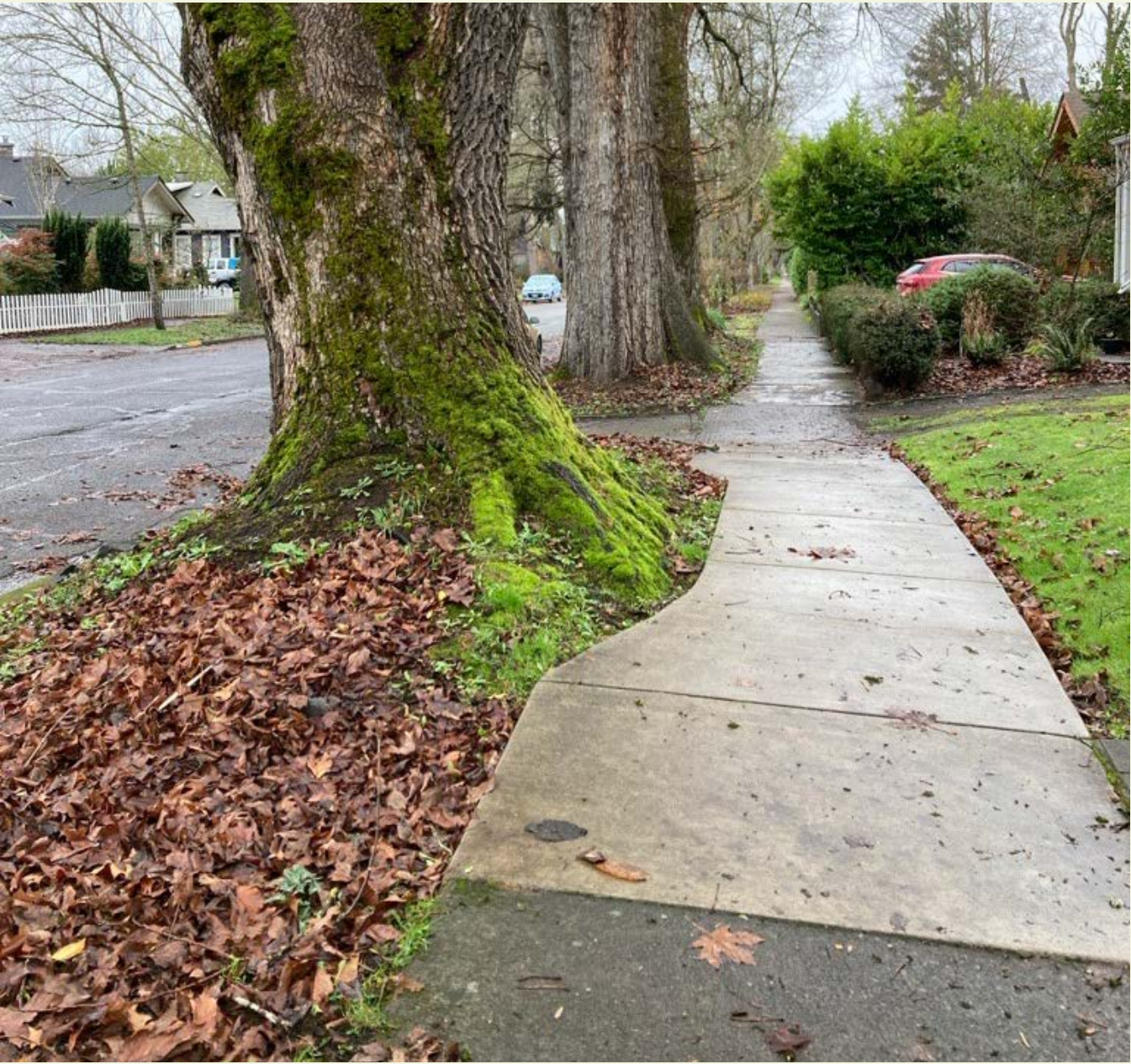
Figure 2.4.15 Example of Modulated Width Photo taken in the field showing one site with a modulated plant bed. Excessive cross slope is perceptible pointing away from the tree.
