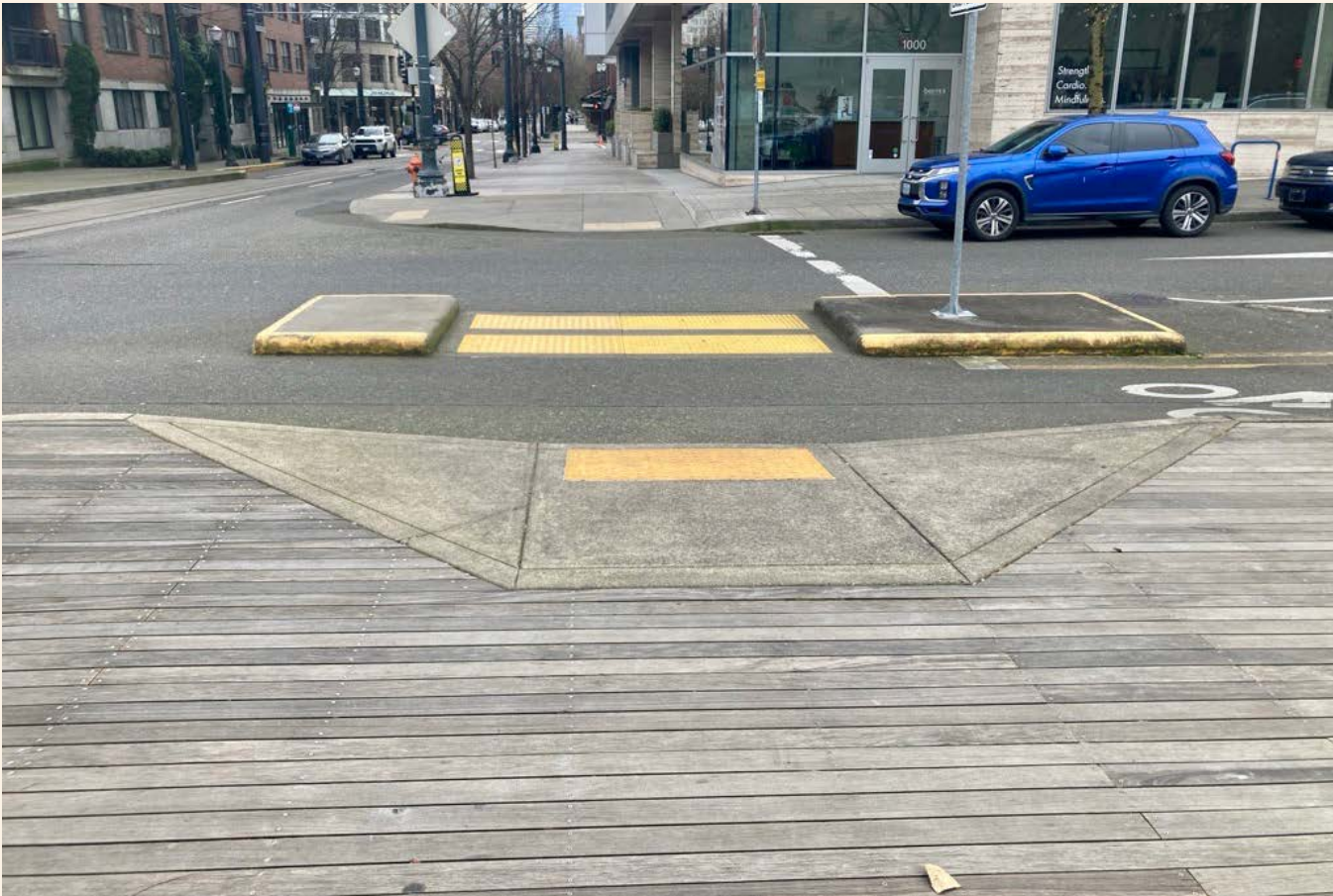
Figure 3.2.6 Jamison Square Curb Ramp Photo demonstrating how the Jamison Square Boardwalk connects to curb cuts.
