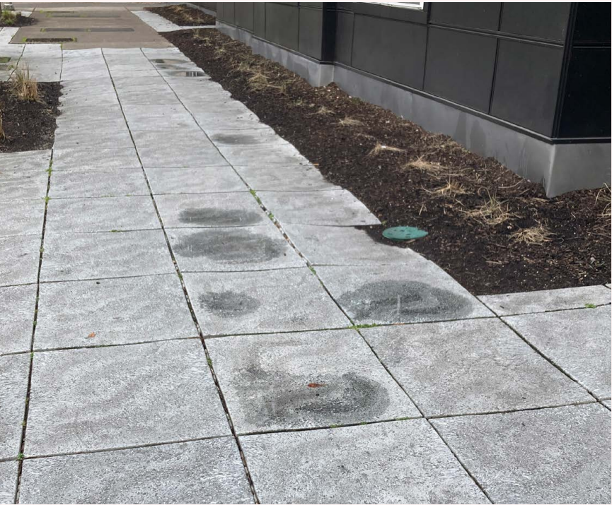
Figure 1.3.14 Water Pooling on Terrewalk System Panels Photo of in-tact Terrewalk system panels with bowls holding water from adjacent irrigation.
