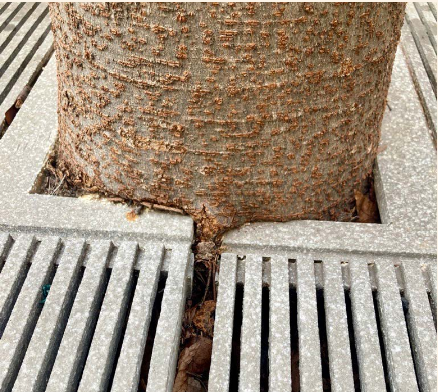
Figure 3.2.7 Jamison Square Tree Grate Photo of a tree grate installed in Jamison Square, demonstrating how the product is constraining the tree’s base.
