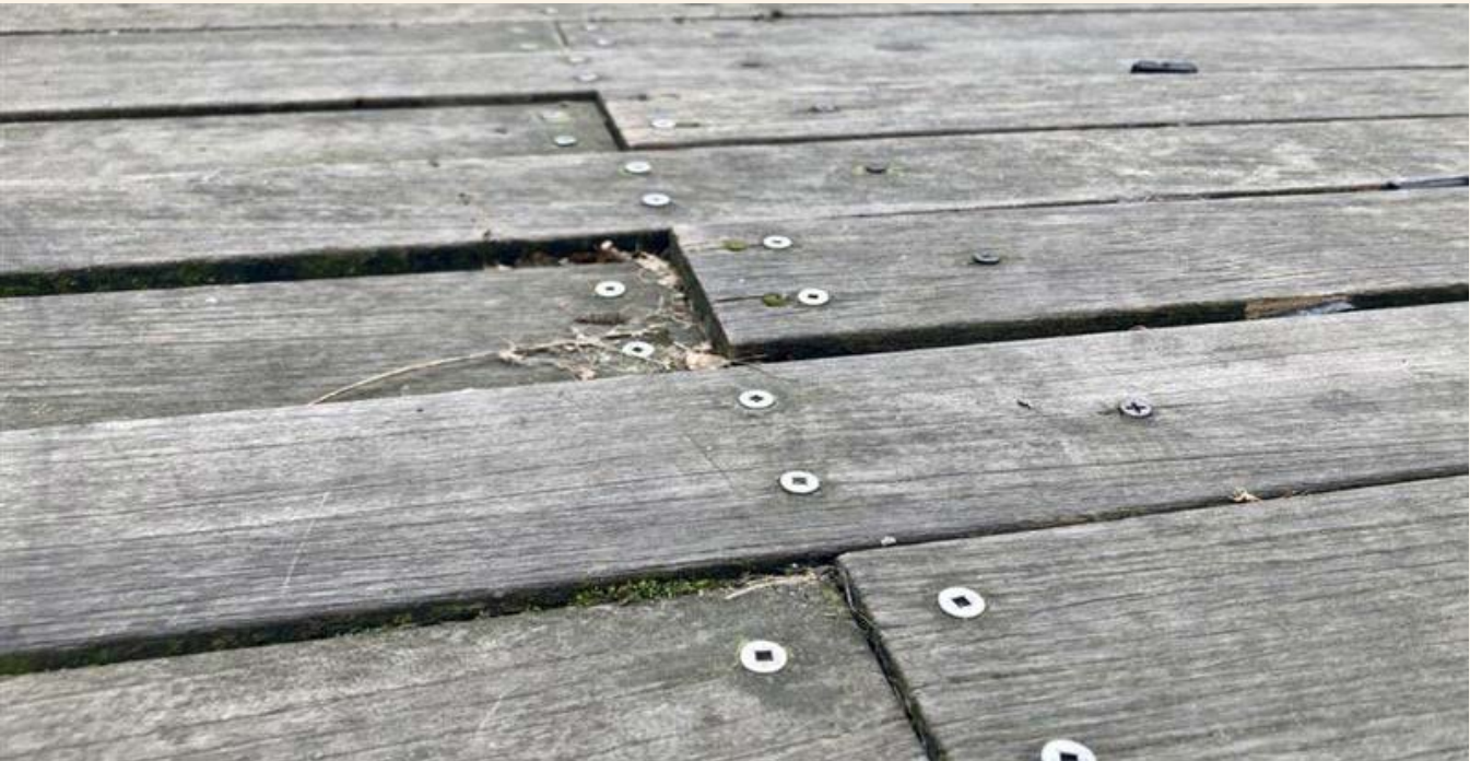
Figure 3.2.5 Jamison Square Wear and Tear Close-up views of the boards at Jamison Square warping, likely through moisture/heat expansion and contraction, causing level changes, and images of sections with heterogeneous age, indicating recent repairs.
