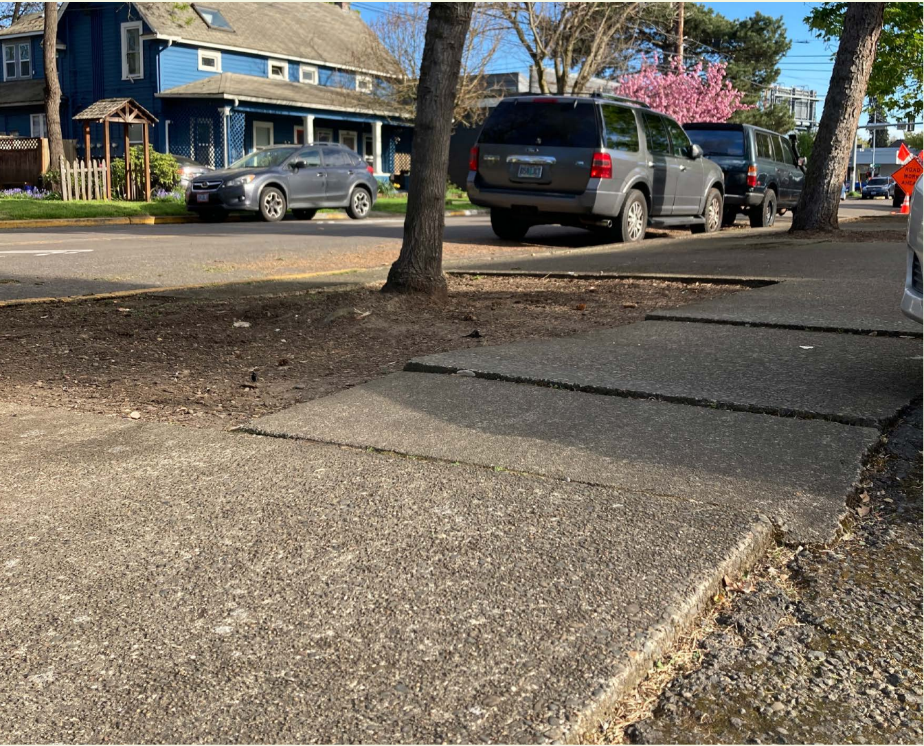
Figure 2.5.3 Small Bigleaf Maple Breaking Adjacent Sidewalk
