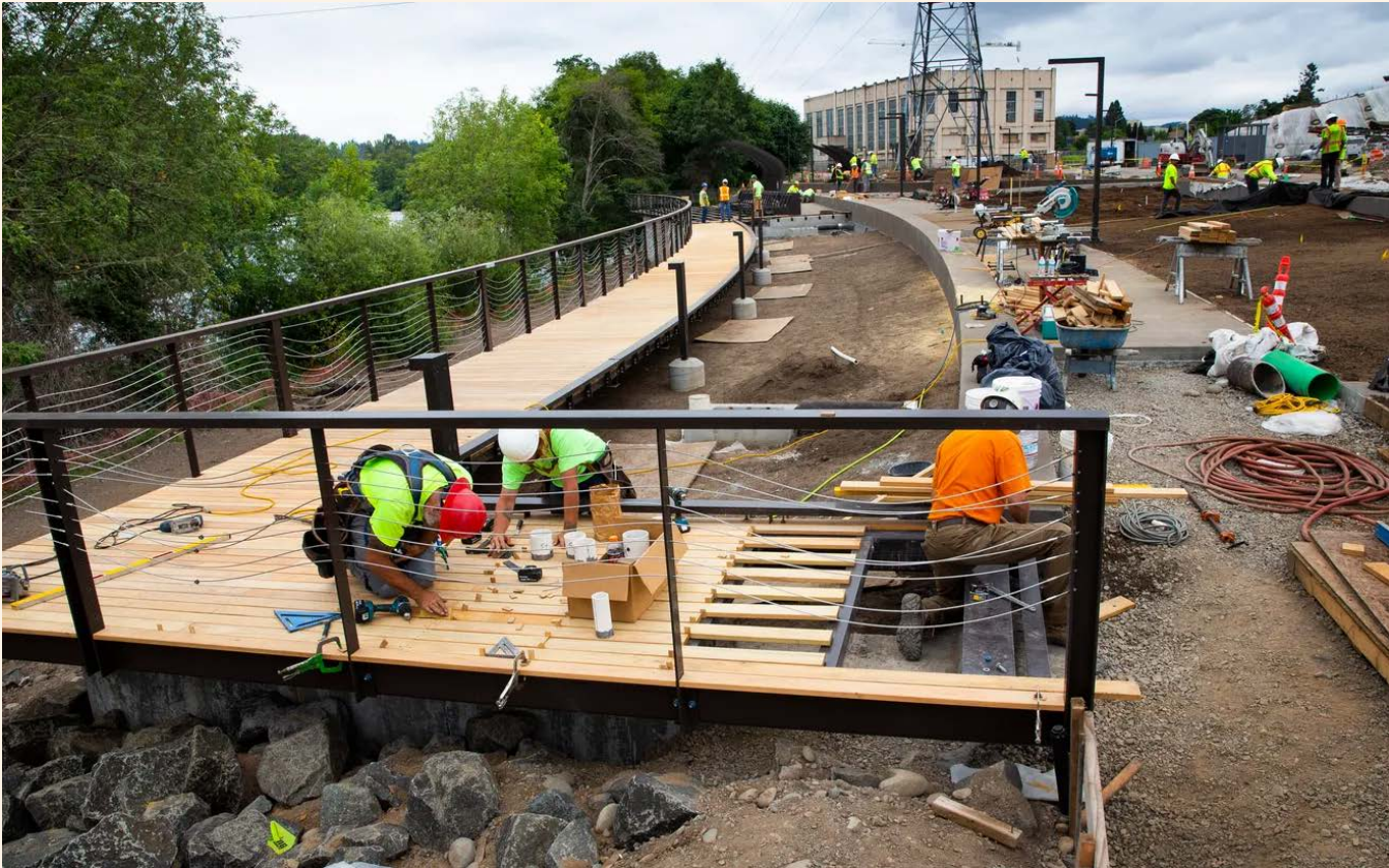
Figure 3.2.2 Downtown Riverfront Boardwalk Photo of the boardwalk along the Eugene Riverfront under construction. (Pietsch, 2021)
