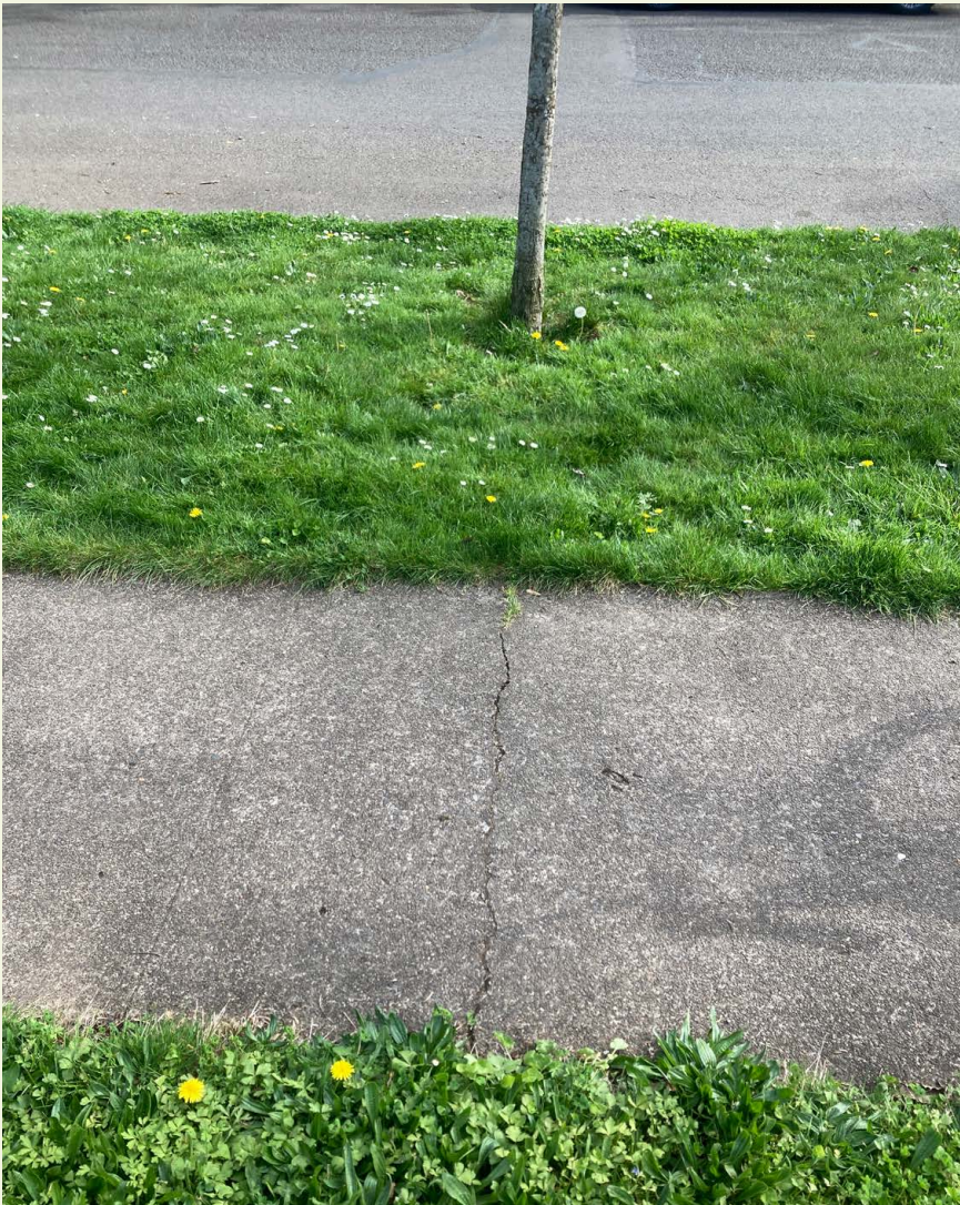
Figure 2.5.2 Small Bigleaf Maple Cracking Adjacent Sidewalk
