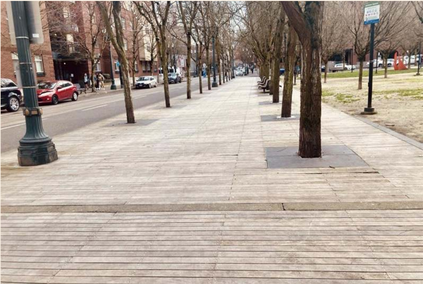
Figure 3.2.4 Jamison Square Boardwalk Wide wooden boardwalk in Jamison Square in Portland, OR. Boardwalk is on-grade and encloses trees with grates. The main circulation route appears even and accessible, but there are some visible level changes along the sides, particularly between tree grates.
