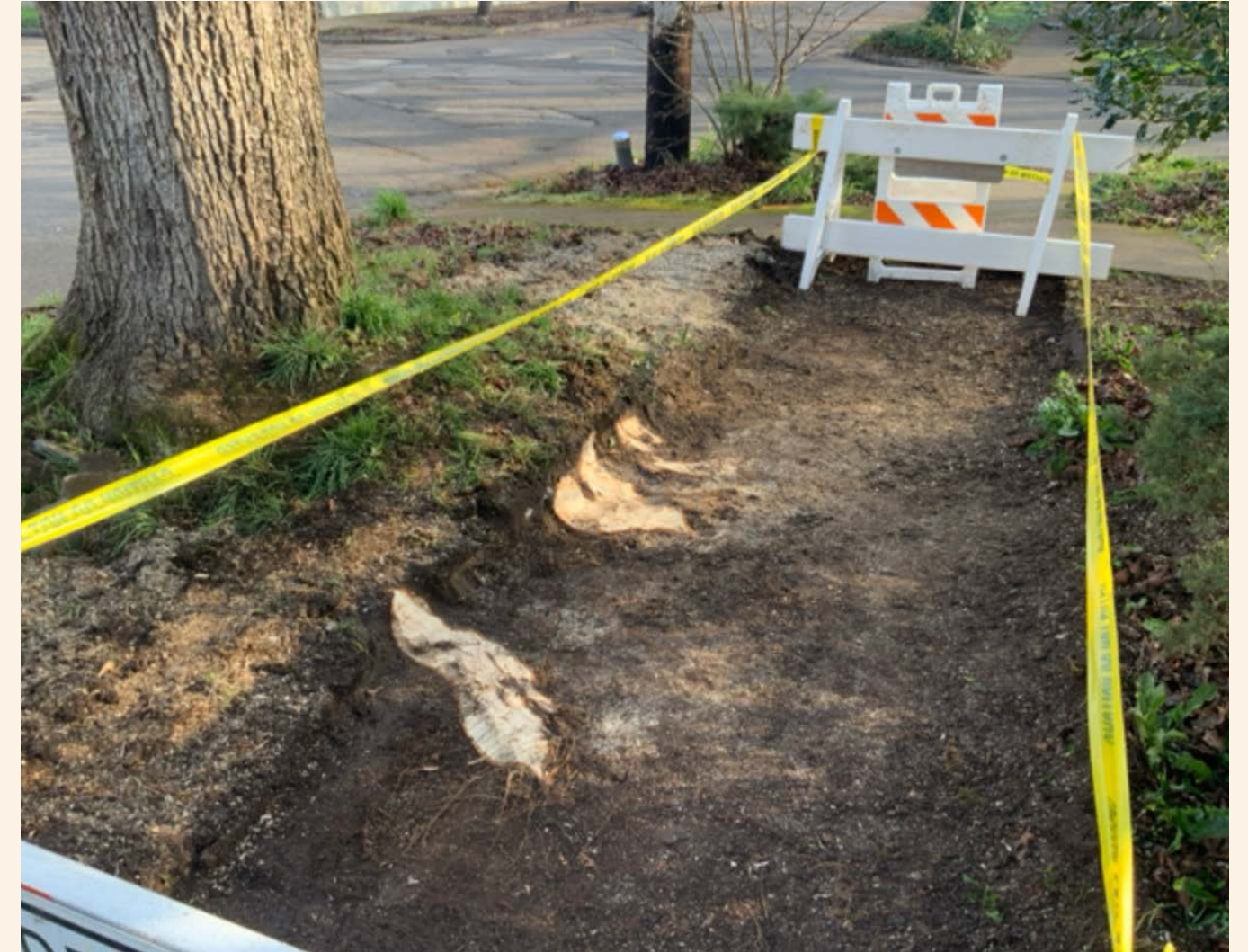
Figure 3.3.12 Root Pruning Required to Save the Smaller Majestic Maple
