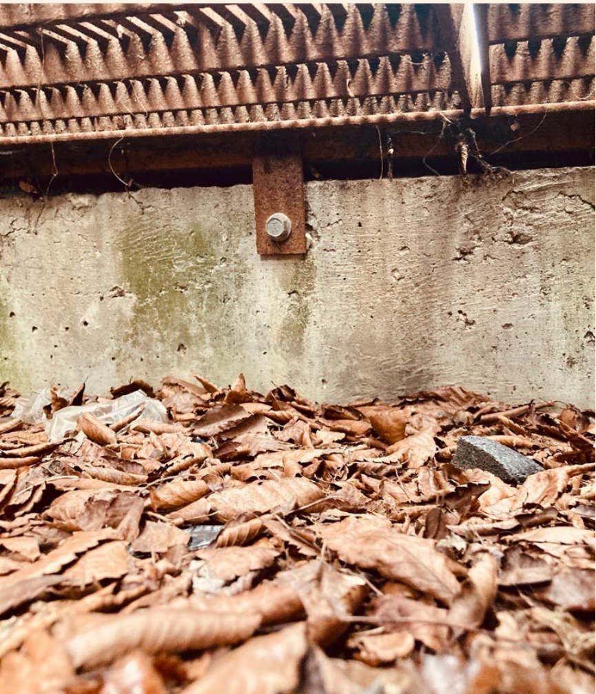
Figure 3.2.8 Inside Jamison Square Tree Grate Photo taken below grade inside of a tree grate, showing that the grates and apparently the boardwalk itself are secured onto concrete beams, which provide some air space between them, but clearly occupy the space trees’ roots prefer to grow, enclosing the trees planted in Jamison Square.
