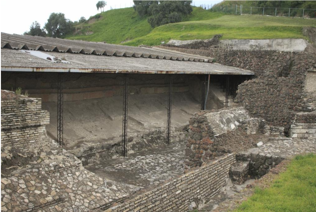
Figure 7: Layers of construction, Tlachihualtepetl , Building 3. Evidence of the Pre-contact tradition of covering over sacred spaces (Photographed by the author, August 2011).
