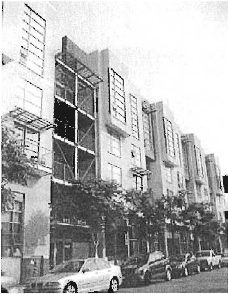
Fig. B.2.c.7. highly articulated facade with projections and recesses signify residential function of the building
