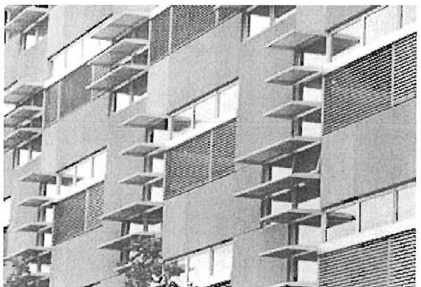
Fig. B.2.c.1 sun shades used to unify the building's street wall and add three-dimensional quality
