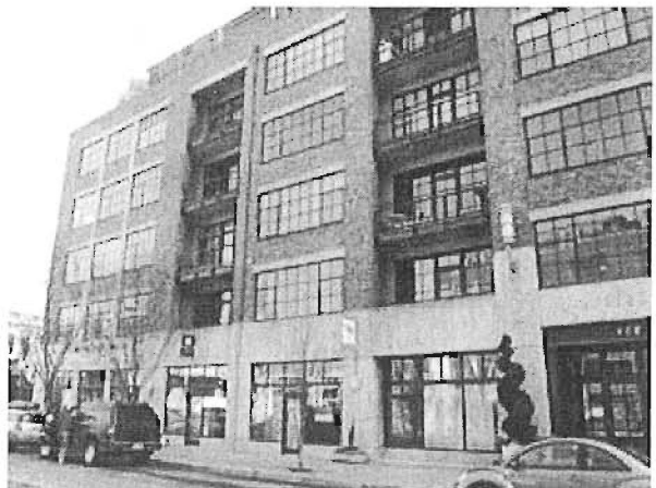
Fig. B.2.c.3. facade components establish the building's clear and pleasing set of proportions
