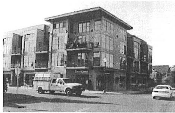
Fig. B.7.c.1 over sized projecting eave highlights an important corner
