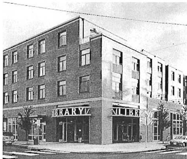
Fig. B.1.c.1 Simple massing emphasizes deep openings that create shadow lines in this "background" building.
