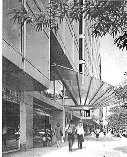
Fig. B.6.d.3 large, distinctive canopy highlights a main entrance
