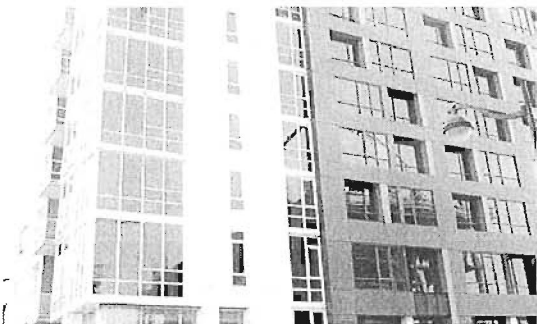
Fig. B.2.c. 8&9. change in fenestration, color and recessed windows animates an otherwise flat facade
