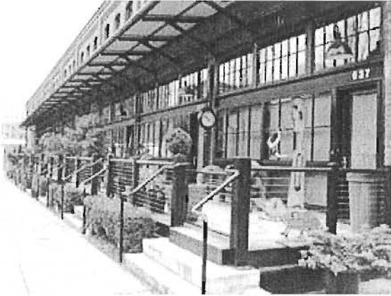
Fig. B.2.c.2.1. former warehouse gets a new life as a residential building
