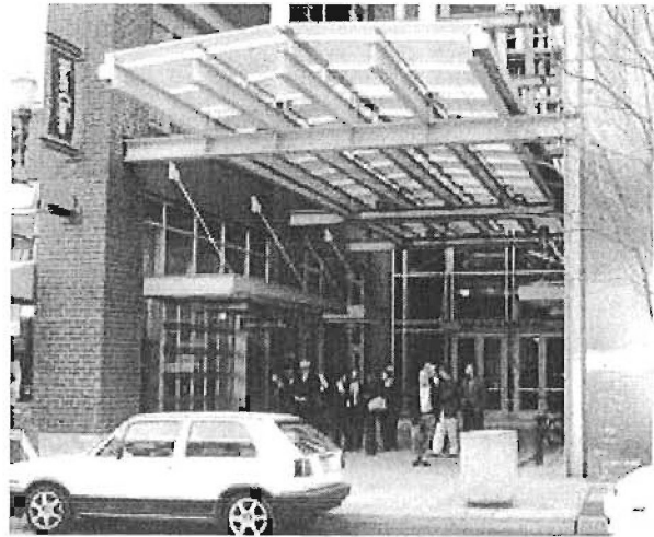
Fig. B.6.c.4 (1) oversized canopy and columns emphasize the main entry
