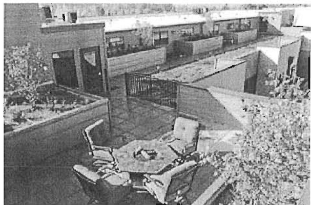
Fig. B.7.c.2 rooftop terrace
