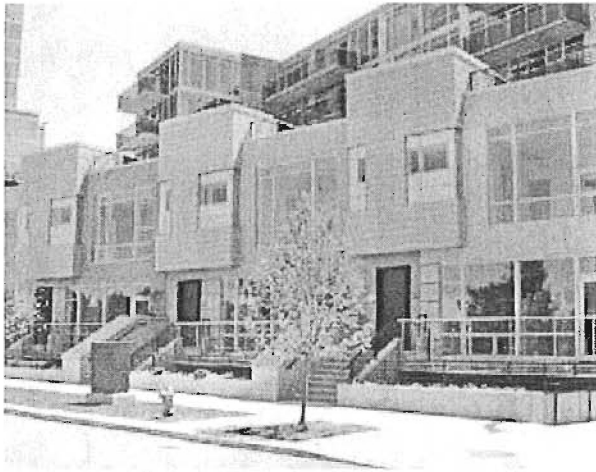
Fig. A.2.c.1 & 2 multiple entries and stoops enliven the street with minor grade separations to protect residential privacy
