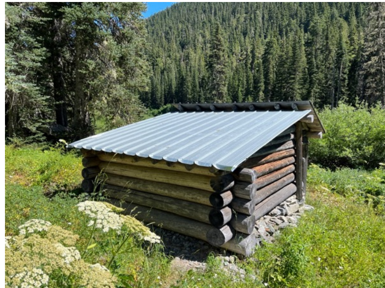
Along with the two shelters at Blue Glacier, Wilder (pictured top row) and Bear Camp (pictured bottom row) are the only remaining shelters of the early post-WWII years stacked log construction design. Built in 1951, Wilder most closely resembles what would be the Foster Plan proposed in 1953. It does not, however, feature a firepit near the entrance. Bear Camp shelter, built in 1952, shows a variation of the rounded stacked log construction with a modified gable roof. Both shelters have undergone extensive preservation due to major structural damage including the choice to replace the original split shake roof on Bear Camp with standing metal seam panels. This was done due to the substantial snow loads common at its location. Photos by author 2022.
