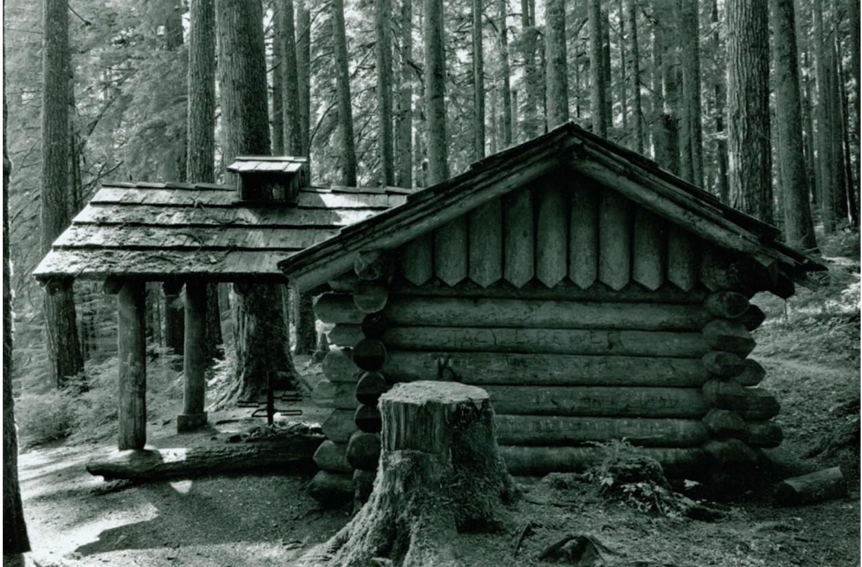
Canyon Creek (also known as Sol Duc Falls shelter) photo dated 1983. Note the concrete blocks supporting the vertical post as well as the firepit with iron or steel cooking rack. Source: Olympic National Park Archives and Collections .
