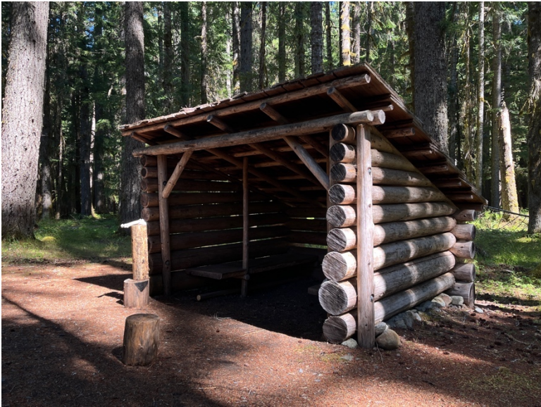
< West and south elevations; note double roof ridge beam
