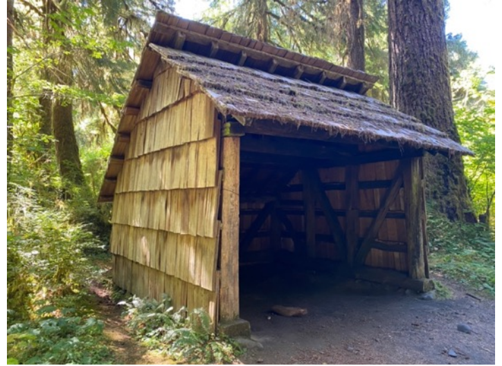
Three Forks (pictured right) shelter, built 1930 and Happy Four (pictured right) shelter, built 1935, are standard examples of the USFS pole and shake Adirondack style. Both are still extant today. Photos by author and Jessica Schmitt respectively.
