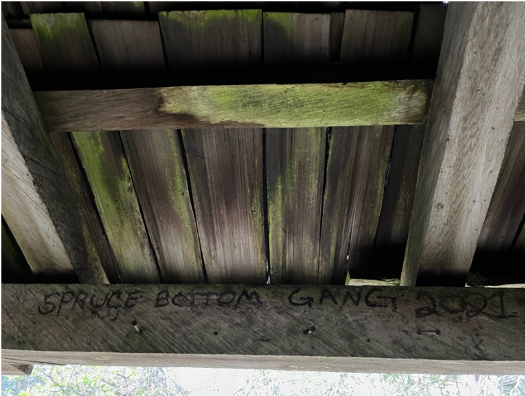
< Example of moisture damage on interior roof structure found throughout
