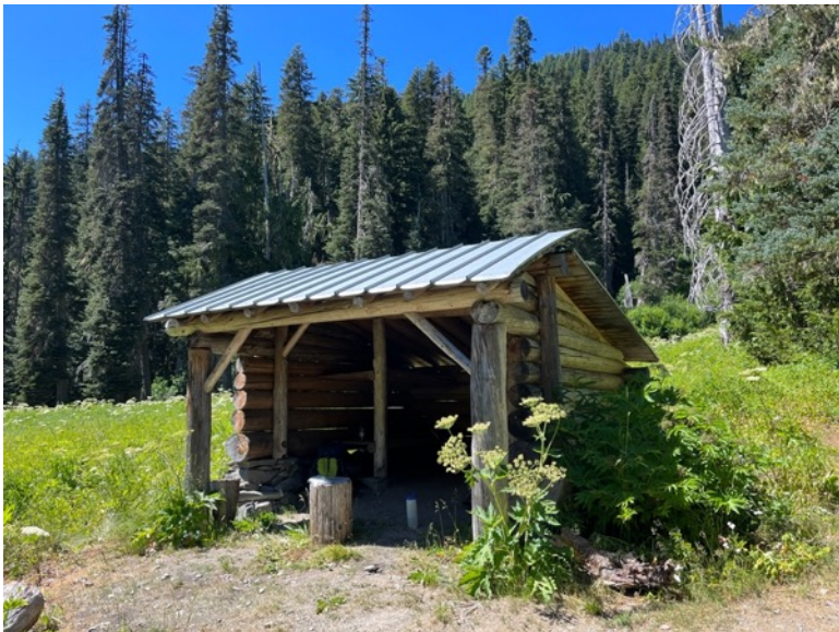
Along with the two shelters at Blue Glacier, Wilder (pictured top row) and Bear Camp (pictured bottom row) are the only remaining shelters of the early post-WWII years stacked log construction design. Built in 1951, Wilder most closely resembles what would be the Foster Plan proposed in 1953. It does not, however, feature a firepit near the entrance. Bear Camp shelter, built in 1952, shows a variation of the rounded stacked log construction with a modified gable roof. Both shelters have undergone extensive preservation due to major structural damage including the choice to replace the original split shake roof on Bear Camp with standing metal seam panels. This was done due to the substantial snow loads common at its location. Photos by author 2022.
