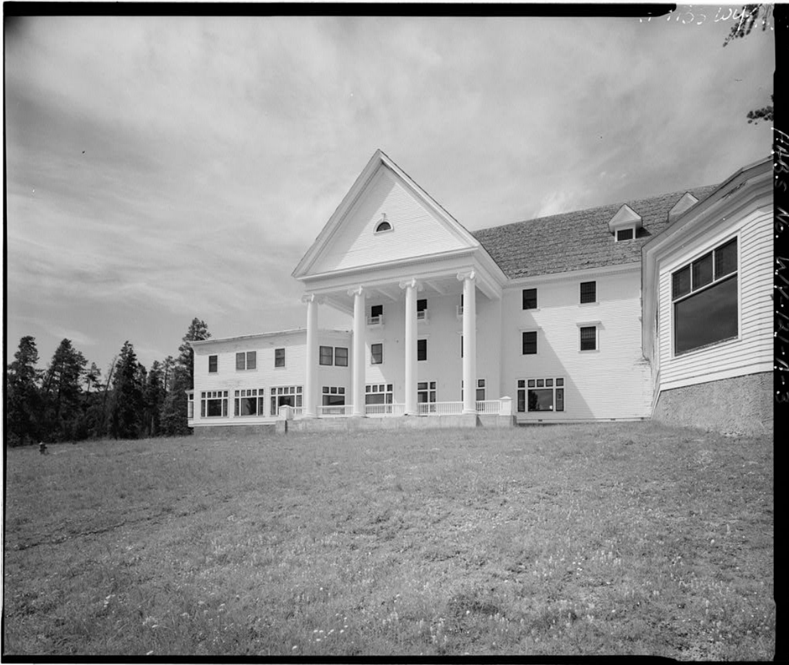
The Lake Hotel was built in 1891 to accommodate visitors of Yellowstone National Park. The hotel was built in a colonial revival style popular at the time. Despite the use of wood, the formalized columns and pedimented gables bear little connection with the wooded natural surroundings, creating a lack harmony between the hotel and the environment. Source: Library of Congress, Prints & Photographs Division, HABS, Reproduction Number: HABS WYO, 20-LAK, 1A-3.
