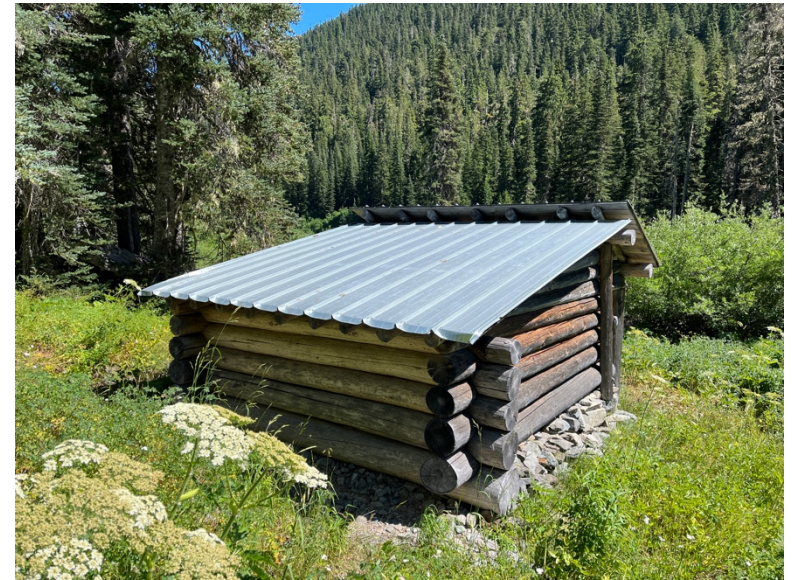
^ North and west elevations showing extent of vegetation encroachment around periphery of building
