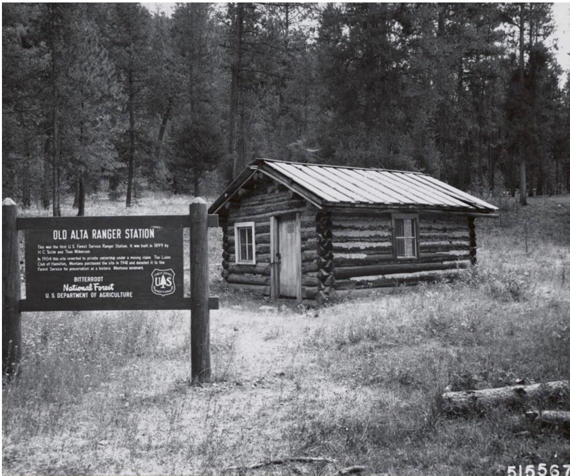
Alta Ranger Station built in 1899—considered to be the oldest Ranger Station in the US—is an example of early vernacular construction built to serve public lands under the Forest Reserve and later USFS. The use of local materials naturally blended into the environment from which they were harvested and would come to inform the “Rustic” architecture popular with agencies such as the USFS and NPS. National Archive and Records Administration. National Archives Catalog. Record group 95: Records of the Forest Service. Series: Photographs Relating to National Forest, Resource Management Practices, Personnel, and Cultural and Economic History. NAID: 7003660
