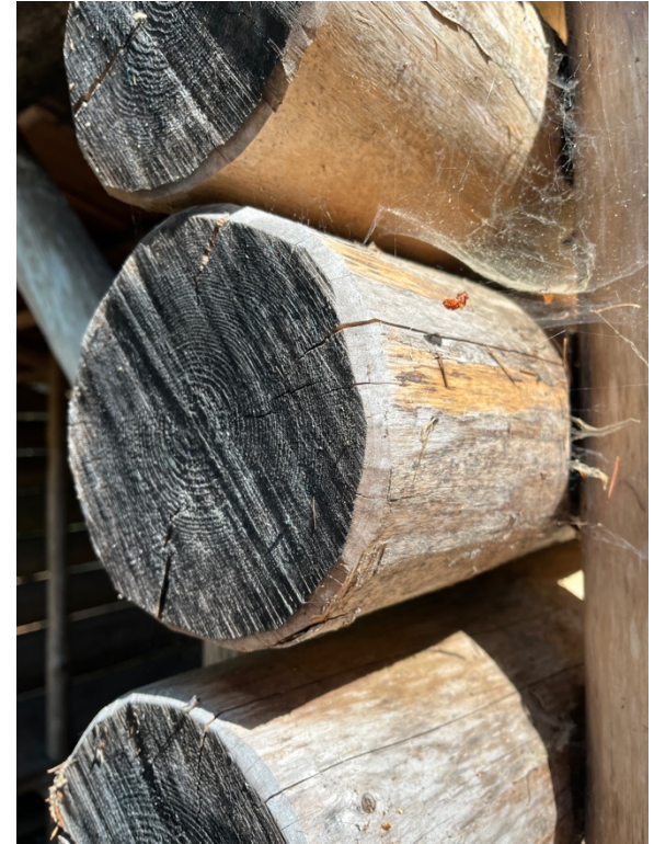
^ Detail of chamfering around log edges
