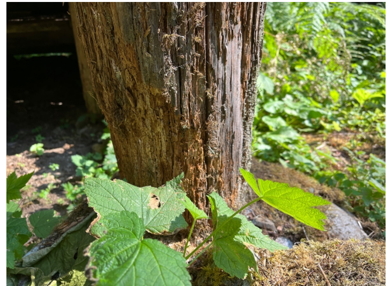
Example of deterioration found at both corner posts >
