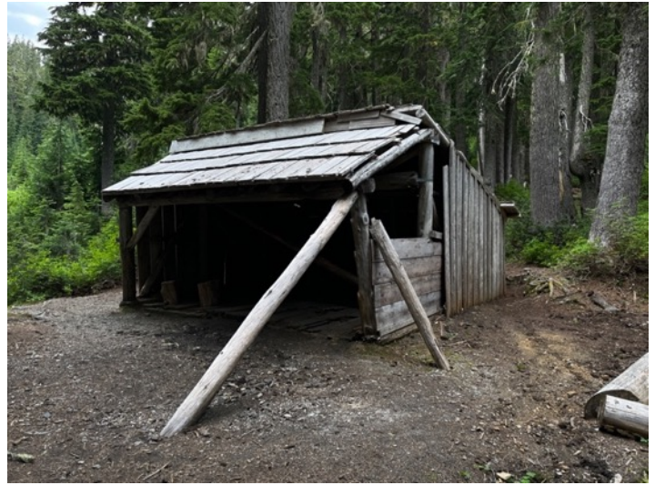
Left: Elkhorn Guard District shelter was built in 1933 as part of the larger Elkhorn Guard District including a ranger station, shed, and horse barn. This shelter has been moved from its original position in the meadow due to the threat of being washed away by the Elwha River. The original shake siding was replaced with board and batten in the 1950s. Photo by author.
