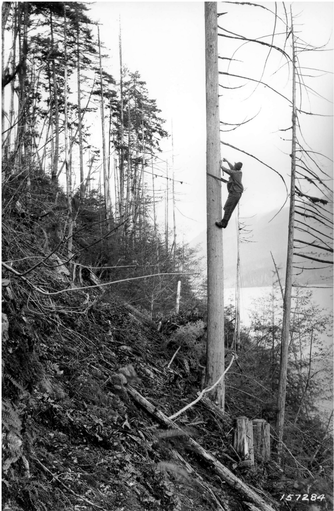
Caption of the photo reads: Ranger hanging [telephone line] insulators Olympic NF WA, 1921. Source: USFS Pacific Northwest Region Archives. Public domain. Digitized online at: https://www.flickr.com/photos/forestservicenw/21416847134/in/album-72157660369045530/
