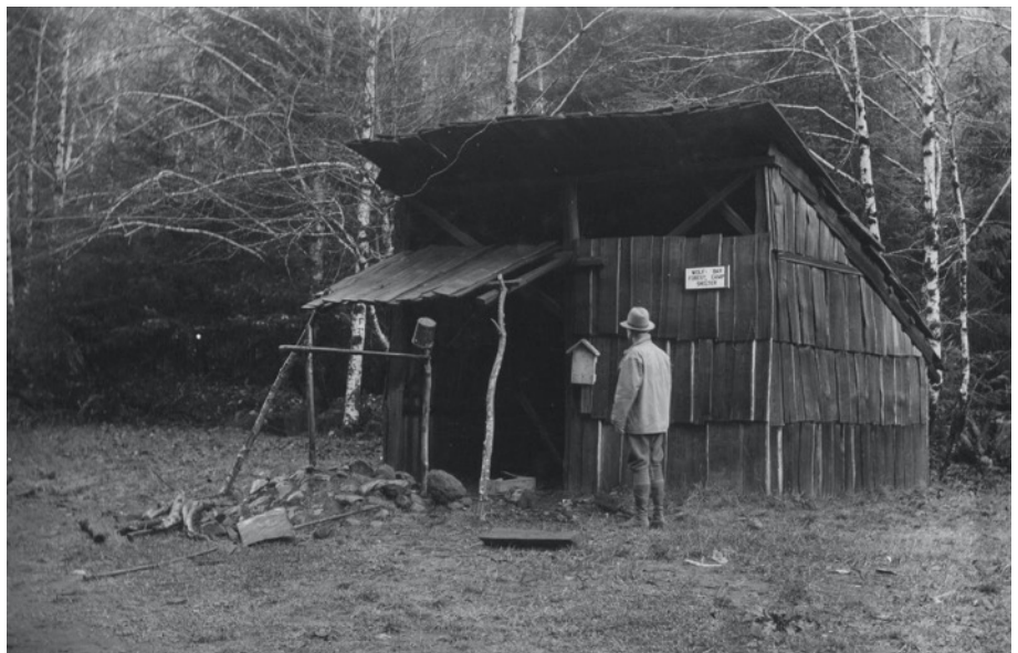
Wolf Bar shelter, construction date unknown. Source: Olympic National Park Archive and Collections.
