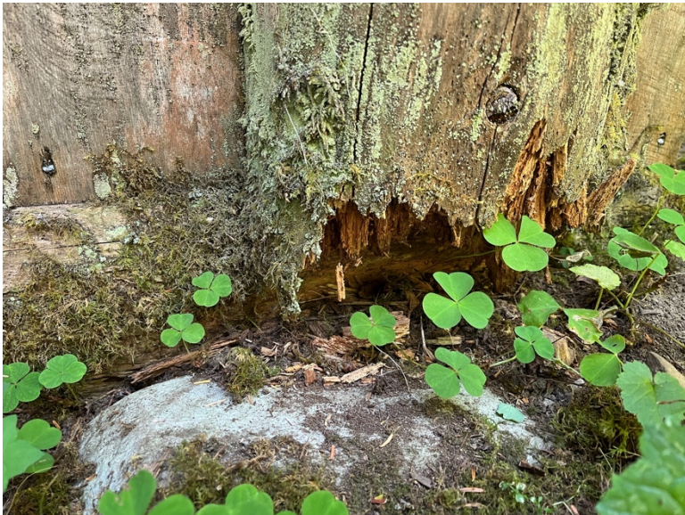
< Detail of deterioration of vertical support posts on north elevation; building generally leaning/ sinking in the NW corner.
