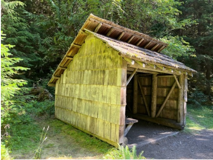
Three Forks (pictured right) shelter, built 1930 and Happy Four (pictured right) shelter, built 1935, are standard examples of the USFS pole and shake Adirondack style. Both are still extant today. Photos by author and Jessica Schmitt respectively.
