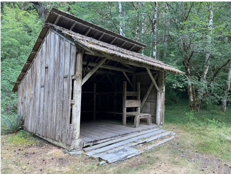
Left: Elkhorn Guard District shelter was built in 1933 as part of the larger Elkhorn Guard District including a ranger station, shed, and horse barn. This shelter has been moved from its original position in the meadow due to the threat of being washed away by the Elwha River. The original shake siding was replaced with board and batten in the 1950s. Photo by author.
