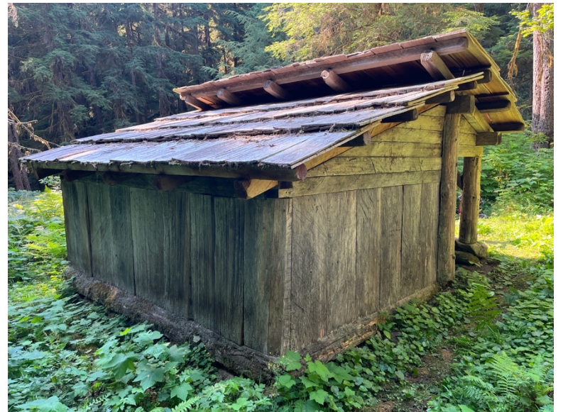
^ East and north elevation showing ground cover encroaching around sill logs
