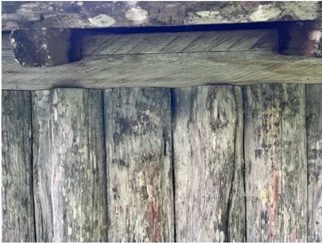
Note: combination of rounded and flat milled wall-log construction. Also note, marks of chainsaw used for milling.
