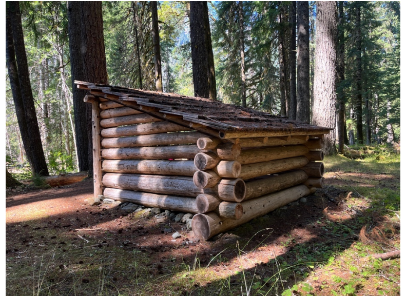
South and east elevations >
