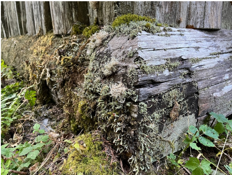
< Detail of organic growth on north and west corner foundation logs; note lap joinery; similar growth along entirety of north, east, and west sill logs
