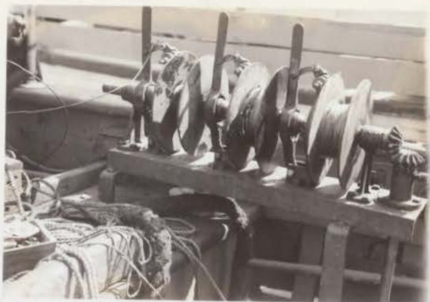
Fig. 3. Gurdies or power reels for hauling heavy trolling lines.
