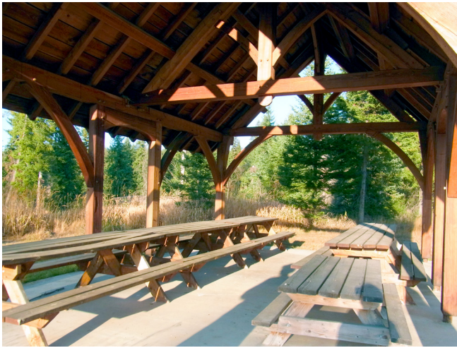
Elk City, ID community center. Photo courtesy of Autumn Ellison, University of Oregon
