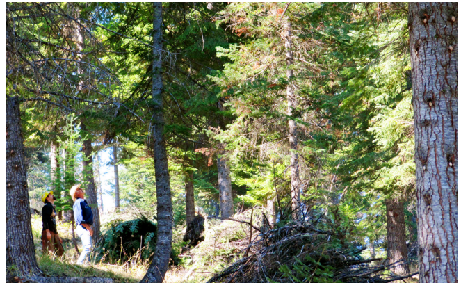
Hazardous fuels reduction work outside of Elk City, ID. Photo courtesy of Emily Jane Davis, Oregon State University.
