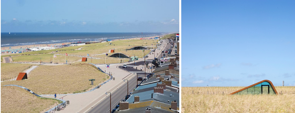
Figure 44. Underground Parking Garage in the Netherlands by Royal HaskoningDHV and OKRA Landschapsarchitecten (2016). From ArchDaily, n.d.
