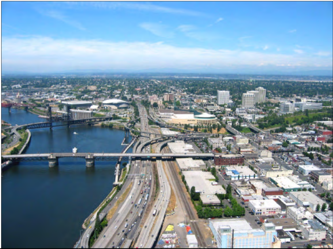
VIEW TO THE NORTH
