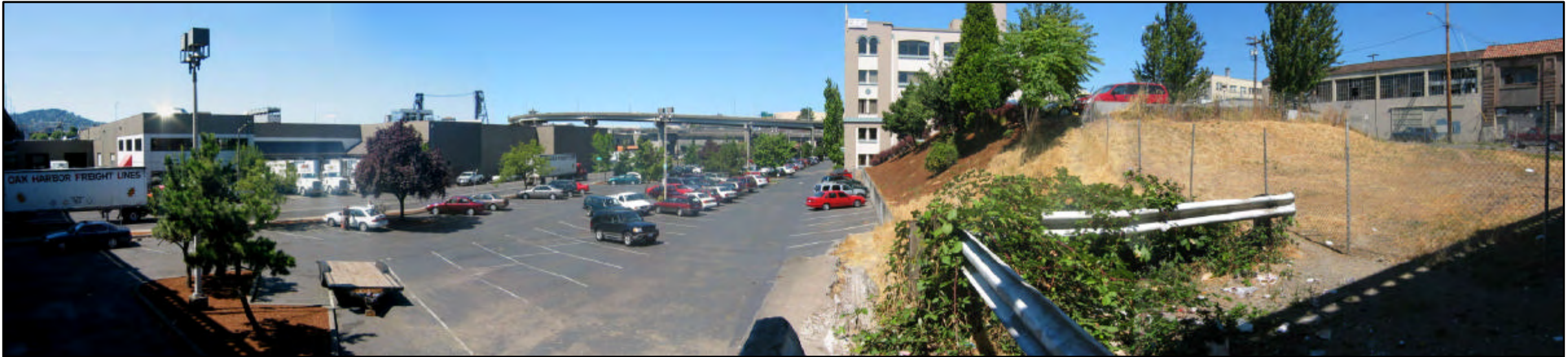
VIEW TO THE NORTHWEST FROM UNDER BURNSIDE BRIDGE
