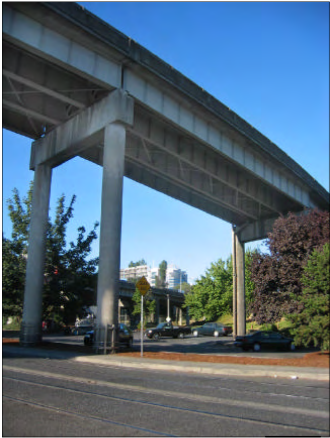
FREEWAY OVERPASS (BLOCK 69)
