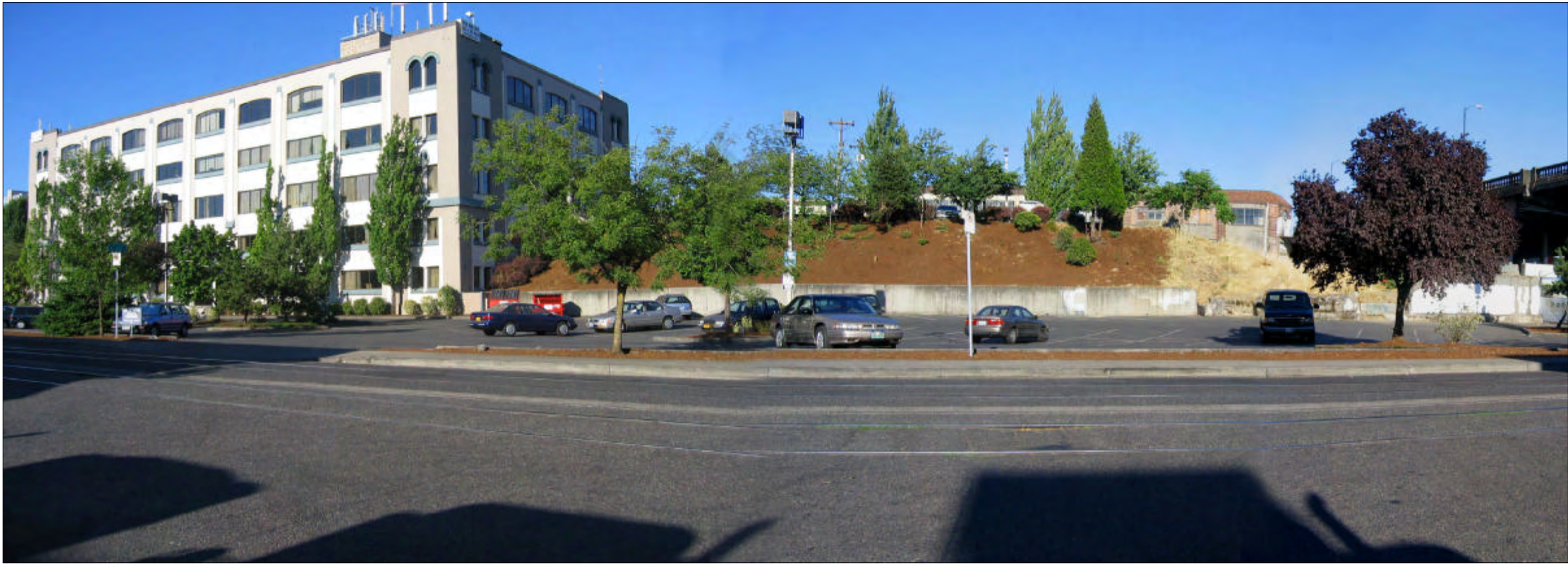
NE 2ND VIEW EAST
