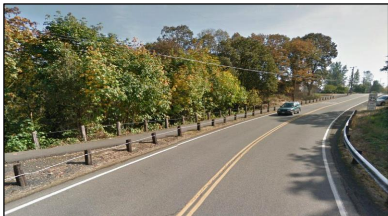
Multi-use, off-street paths like this one on 15 th St can help extend park service areas by providing a comfortable off-street experience
