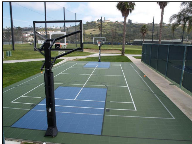
Multi-sport basketball court installation
