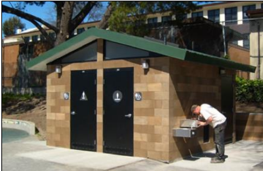
2-stall restroom installation with wall-mounted drinking fountains
