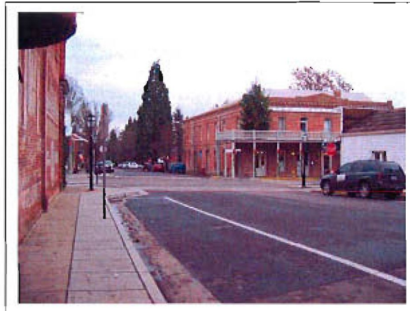
OR 238 (California Street) @ 3rd Street: Looking north through intersection along west side of 3rd Street.
