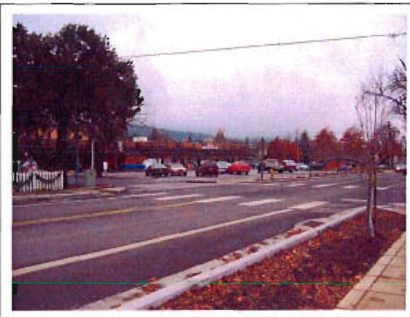
OR 238 (5th Street) @ E Street: Looking northwest through intersection from southeast corner. Jville07.jpg
