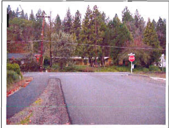
California Street @ 8th Street: Looking south into intersection from north leg (8th Street).
