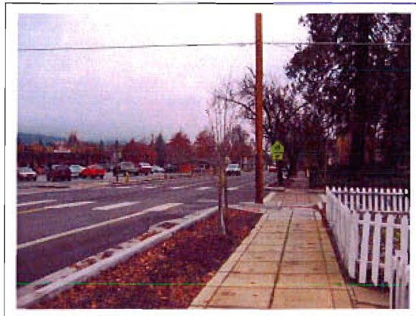
OR 238 (5th Street) @ E Street: Looking north through intersection along east side of 5th Street. Jville08.jpg
