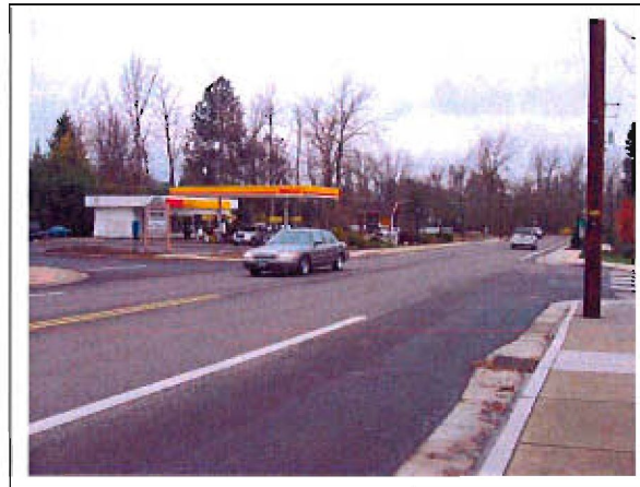
OR 238 (5th Street) @ Shafer Lane: Looking northwest through intersection from southeast corner.
