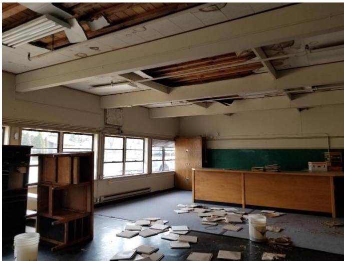
Figure 1: Current condition of one of the classrooms, 2025
