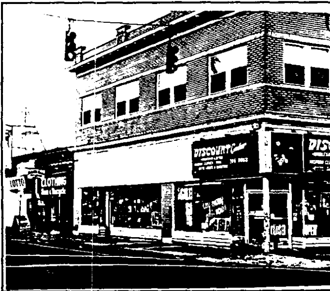
Commercial, institutional and residential uses create an active area at Albina and Killingsworth Streets.
