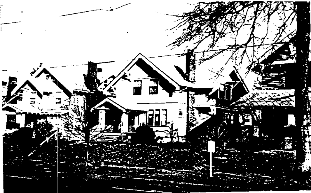
Example of repeating roof slopes.
