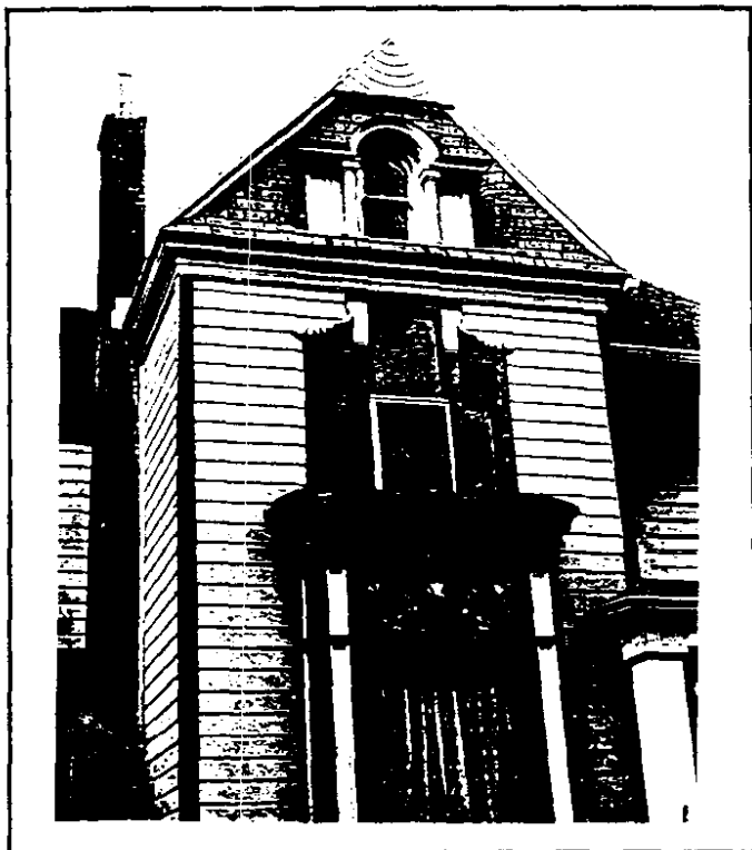
Gable detail with ornamental windows
