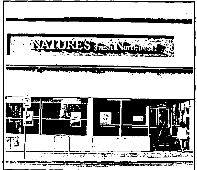
A wall sign such as this at a NE Portland produce and grocery market complements the character of the building.
