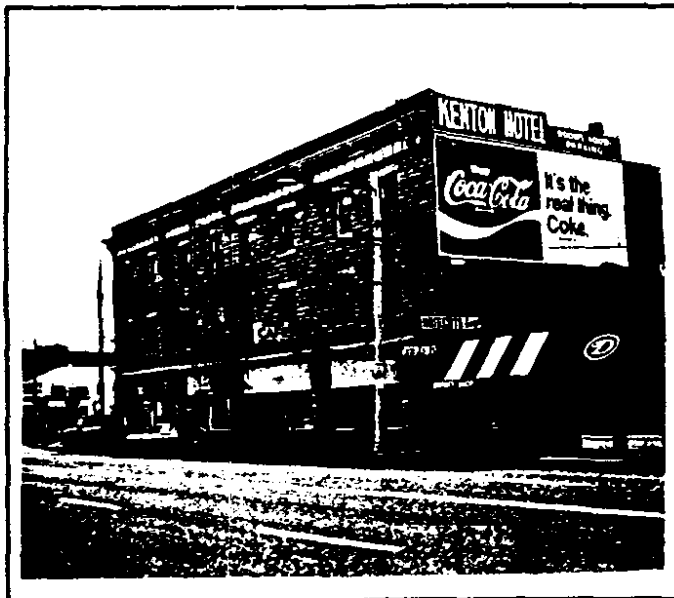
The Kenton Hotel located on N Denver Avenue is a designated historic landmark.
