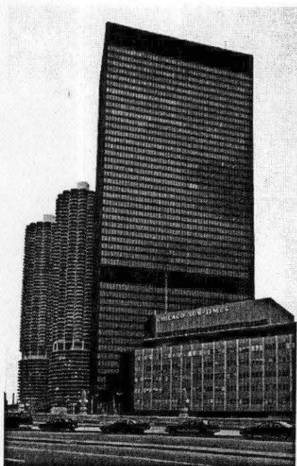
FIGURE 12. I.B.M. Building. (Source: Cohen, 117.)
