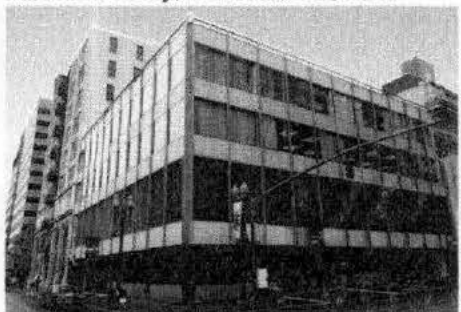
1.15 Glass & Steel Lowrise (+) "float" US MotorBank, Portland, OR, 1954
