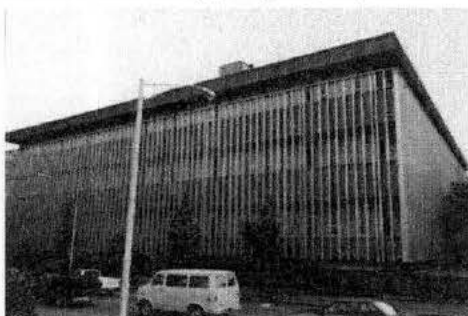
1.12 Glass & Steel Lowrise (+) Lane County Courthouse, Eugene, OR, 1958
