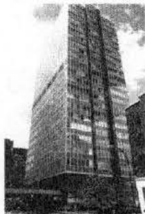
1.21 Glass & Steel Highrise (+) "floater" Guinness Tower, Vancouver B.C., 1967
