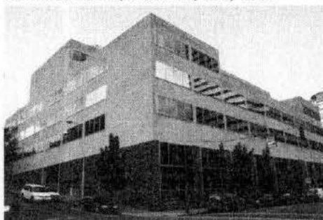
1.16 Masonry (-) Oregonian Bldg., Portland, OR, 1942
