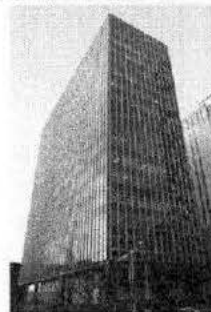
2.15 Glass & Steel Highrise (+) "float" Norton Bldg., Seattle, WA, 1959
