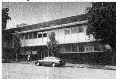
2.16 Masonry (-) Northrup Center, Portland, OR, 1956
