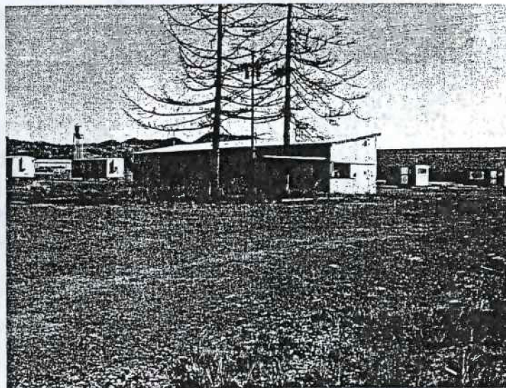
Existing empty structures on TL 400
