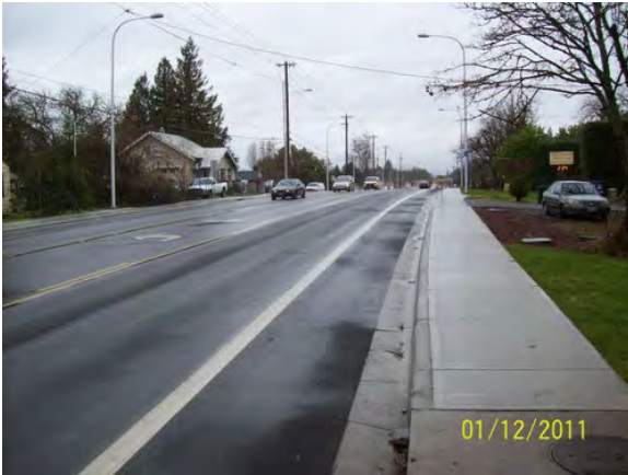
Washington County expanded 185 th Avenue to 3 lanes with sidewalks and bike lanes in an established area of Aloha. Planter strips were not included due to right-of-way constraints.
