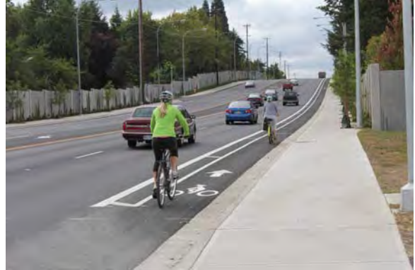
Buffered bike lane on NW 185th Avenue.
