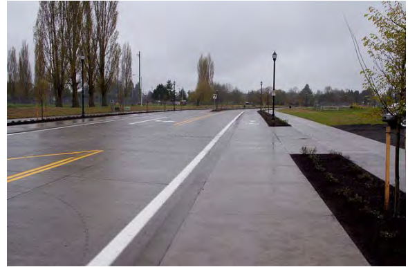
Veterans Drive has a raised cycle track, which was constructed as a joint project between the City of Hillsboro and Washington County at the Fair Grounds.
