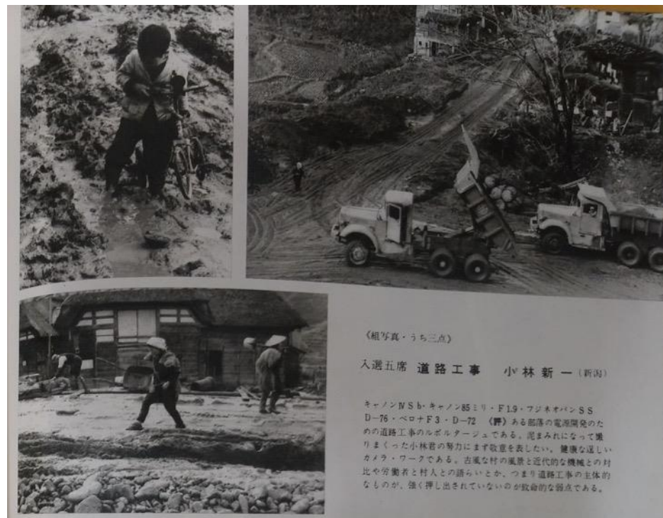
Figure 3.2. Kobayashi Shinichi. “Road Construction” (Dōro kōji). Kamera , March 1955.
