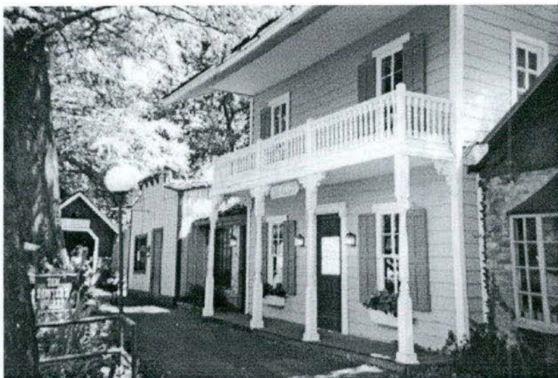
Figure 7. San Marcos Springs, South Bank Shop Facades (photo by author).
