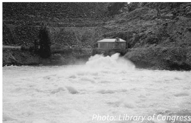
Photo: Library of Congress Downstream face of Tieton Dam
