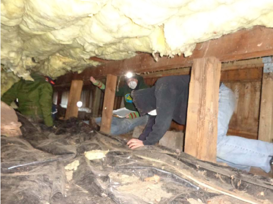
Figure 5.2. Teamwork in the crawlspace of the Briggs House.
