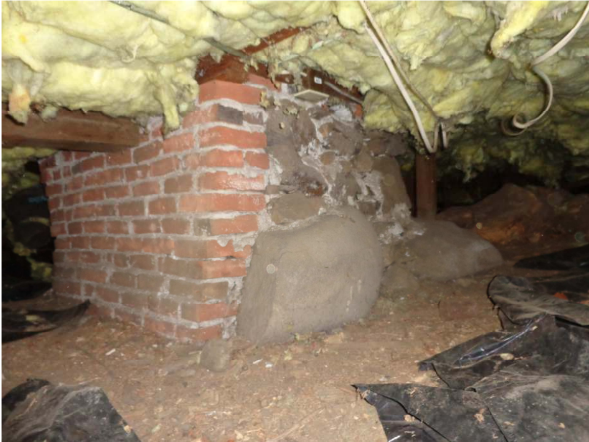
Figure 1.5. Brick chimney foundation built up on base of boulders.
