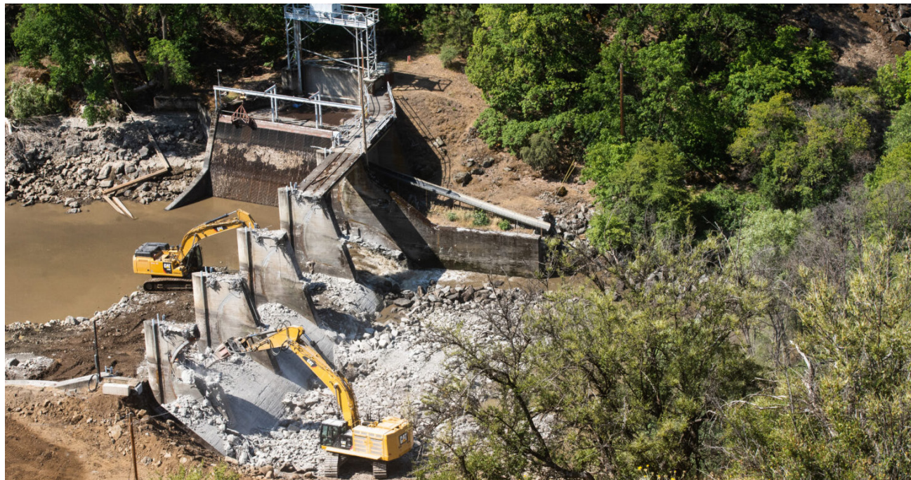
Copco 2 dam removal on the Klamath River, California. Swiftwater Films. 2024. https://www.americanrivers.org/2024/05/four-things-to-know-about-the-impacts-of-dam-removal-on-the-klamath-river/
