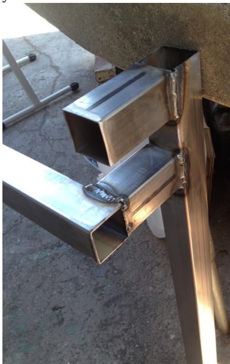
P26. A custom frame to receive the seven luminaires was custom fabricated.
