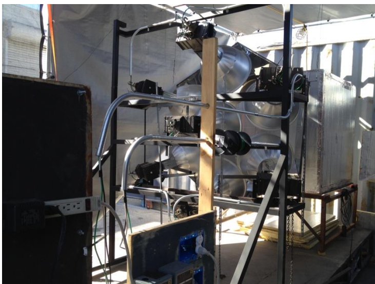
P18. Seen from behind electrical conduits running between electrical panel and each luminaire.
