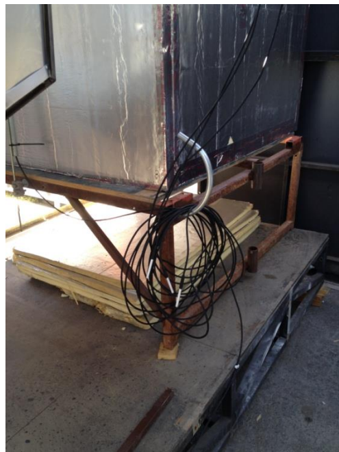
P31. Sensor Hub bundled and ready for deployment as needed
