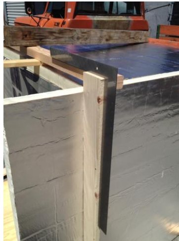
P4. Temporary wood frame used to retain right-angle cube
