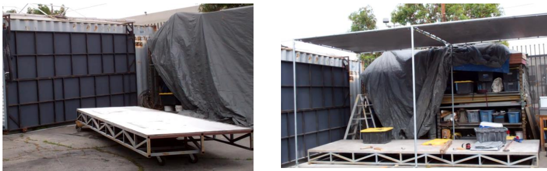
Figure 110: Metal Framed Deck & Canopy
