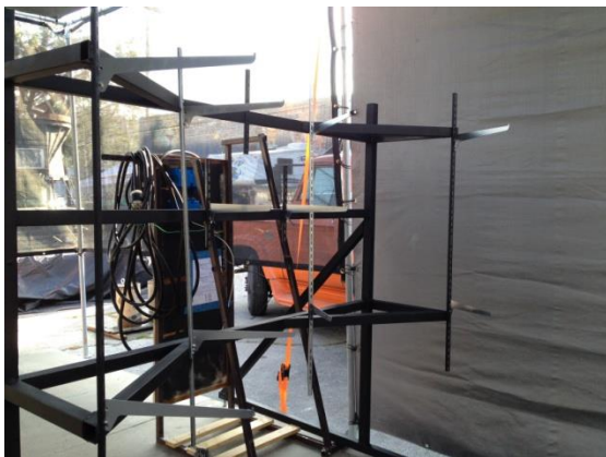
P28. Array frame in place on the metal deck and under canopy.
