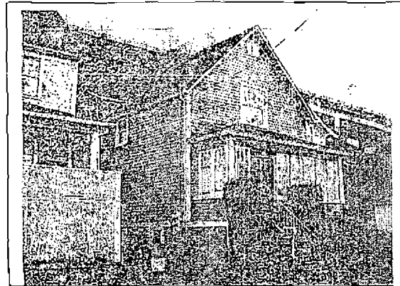
319 W Marine - existing SFD in commercial zone could not be rebuilt if destroyed due to commercial zoning
