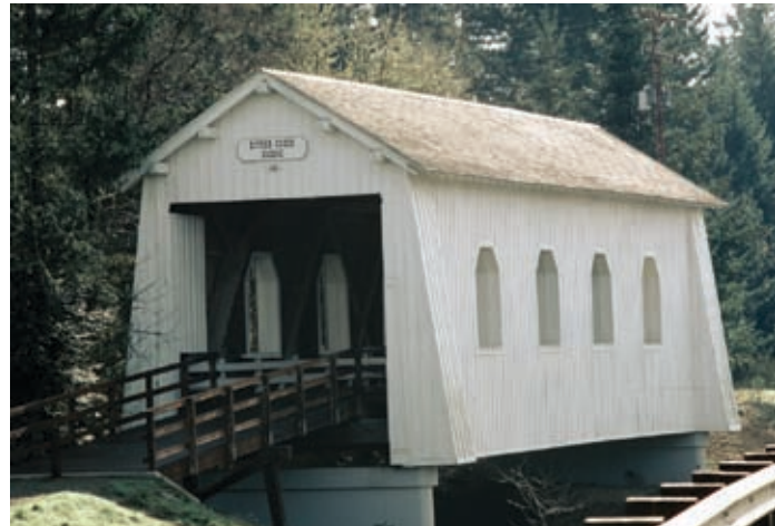
Ritner Creek Covered Bridge, Pedee, Oregon, built 1927
