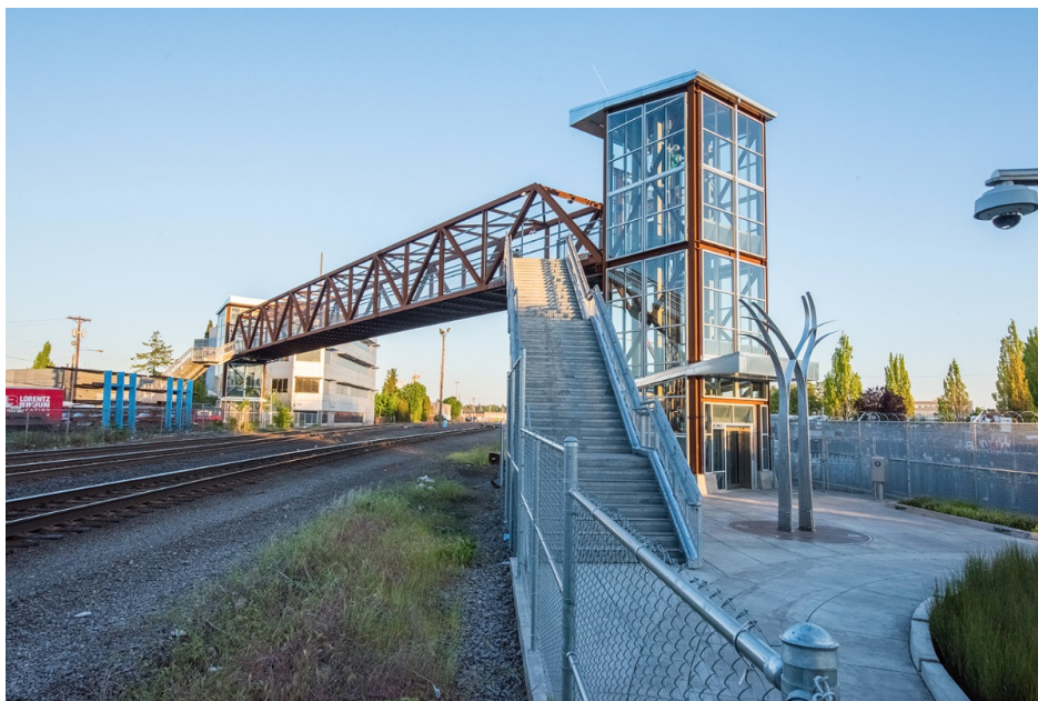
Figure 3.1.1: The Lafayette Pedestrian Bridge, Portland OR (KPF Consulting Engineers, 2021)
