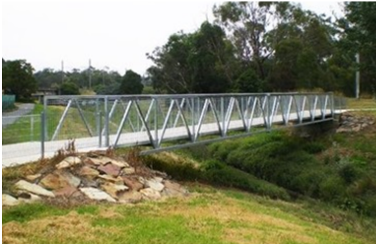
Figure 2.1.2: Steel Truss Pedestrian Bridge (Architecture & Design, 2008)
