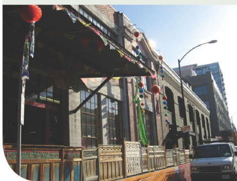
13th Avenue Historic District
