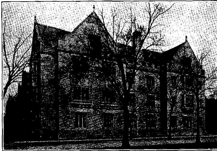
Classics Building, University of Chicago. Built of Gray Indiana Limestone
