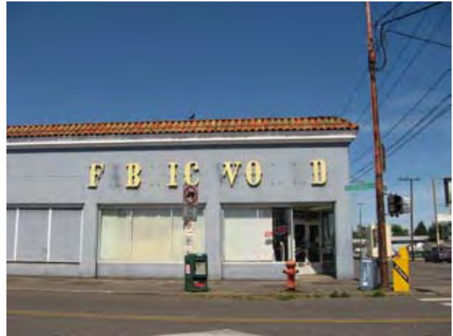
Fabric World is an established business on Lombard with a sign that could use a lift. The business could benefit from a sign and façade improvement program.
