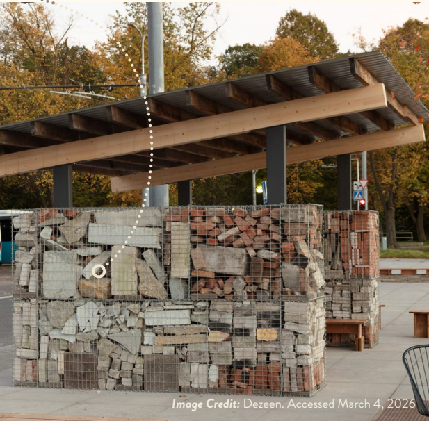
“No Time to Waste” by Brasebin-Terrisse, Tallin, Estonia (2024): A bus stop pavillion built from construction demolition rubble-filled gabion cages with reused corrugated metal roofing and wooden beams.
