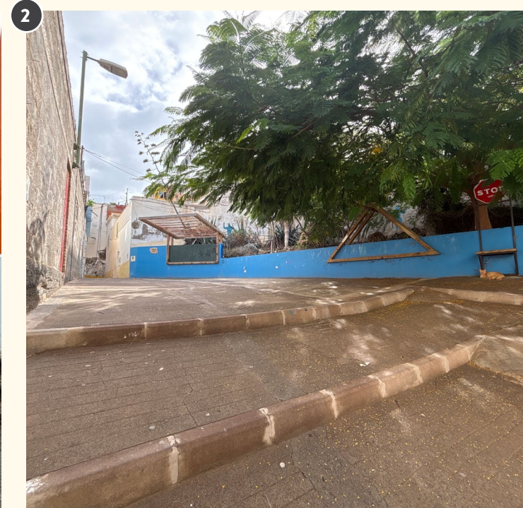
△ Neighborhood Park: Improved as part of the Arquitecturas Colectivas initiative, this once vacant lot is now one of El Risco’s most vegetated public spaces.
