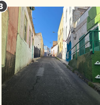
Narrow corridors with little direct sunlight ever reaching the groundplane.
