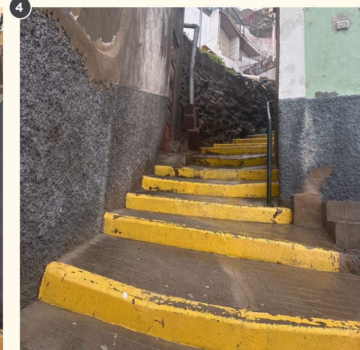
△ Narrowing: Double-wide steps shrink to single-width pedestrain access as circulation snakes through buildings.
