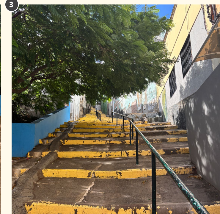
△ Escaleras: Step-ramp style staircase retrofitted by neighbors with asphalt between risers to allow for wheeled ascent.
