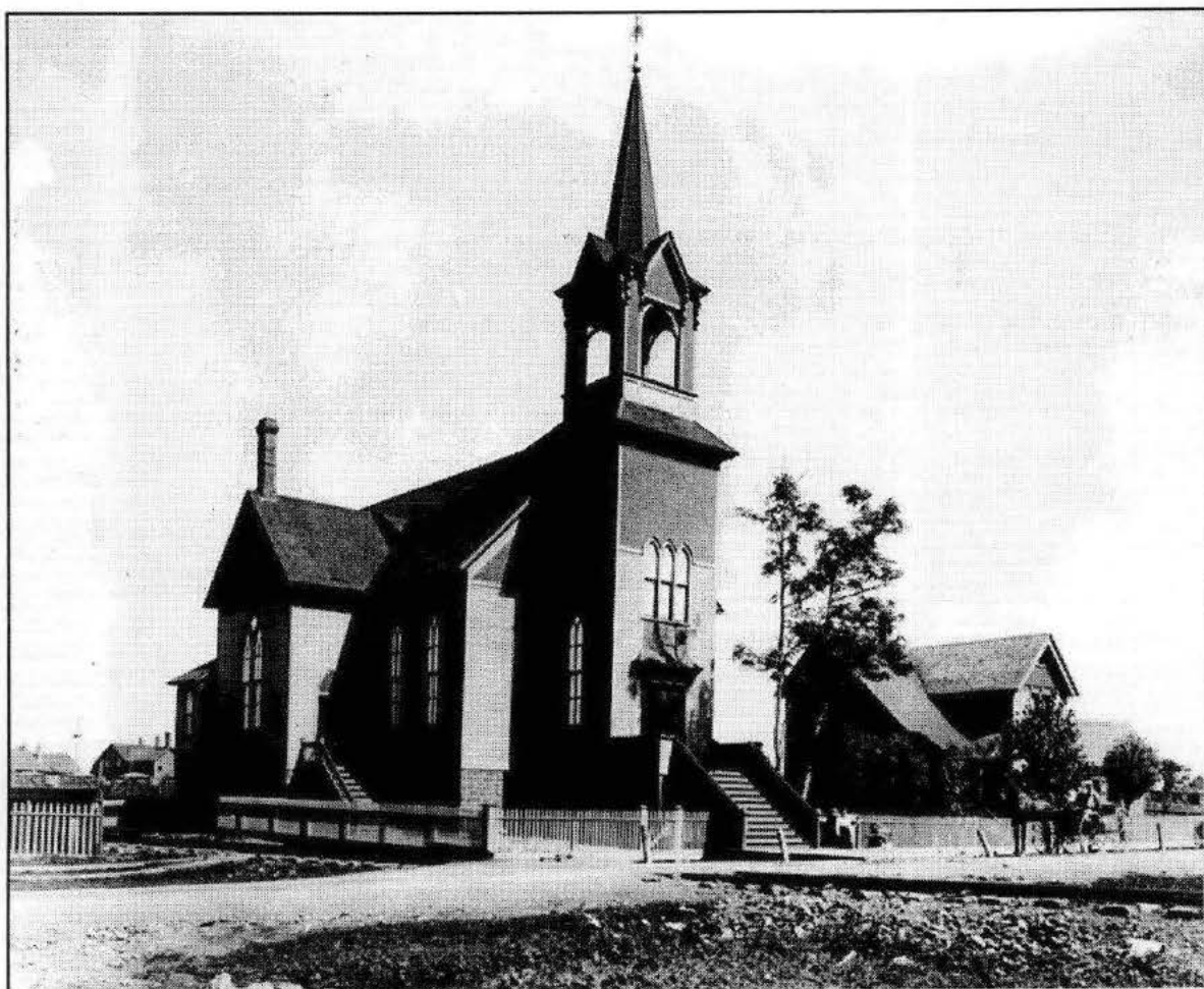
Figure 29. Bethlehem Lutheran Church, Destroyed by Fire. (Courtesy of the Michigan Technological University Archives and the Copper Country Historical Collections.)
