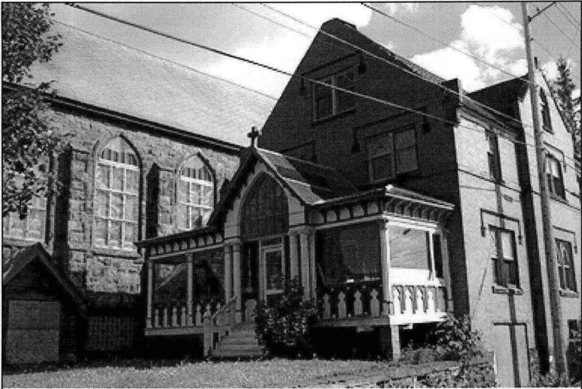
Figure 4. Facade of St. Anne's Rectory with the Church in the Background.
