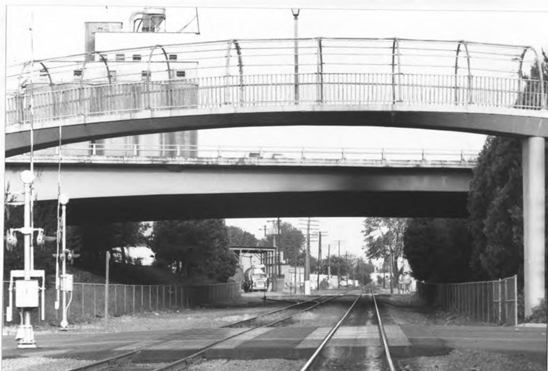
Figure 18: This photograph illustrates the complexities involved in moving trains and automobiles through the same places. The Eugene city street in the foreground is fit to the rails with special inserts which allow locomotive wheels to pass unimpeded. It is also guarded by crossing gates, two of which are visible on the far left. The bridge in the background lifts six lanes of freeway over the tracks; the foreground bridge is for pedestrian traffic.
