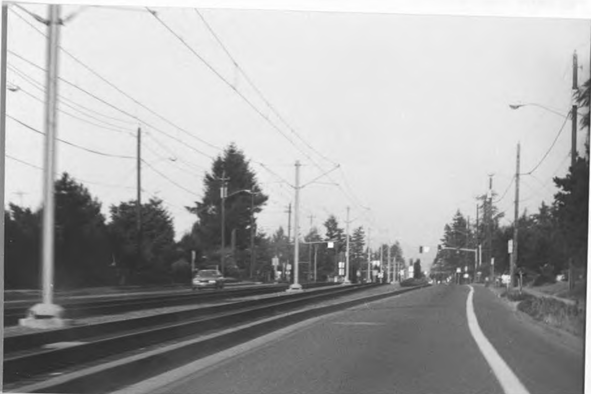
Figure 34: The wires and barricades of the MAX line of Portland's East Burnside Street impose barriers to vision and to automobile movement.
