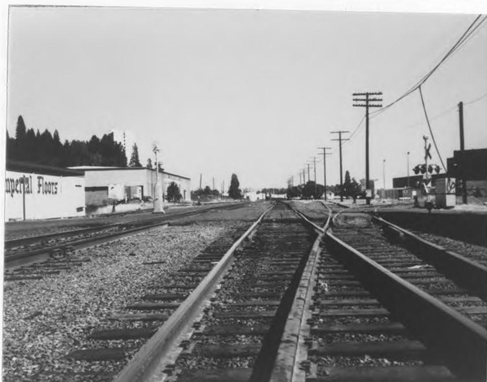
Figure 17: The rail corridor in Eugene is more than half a block wide as it skirts the city's central business district.
