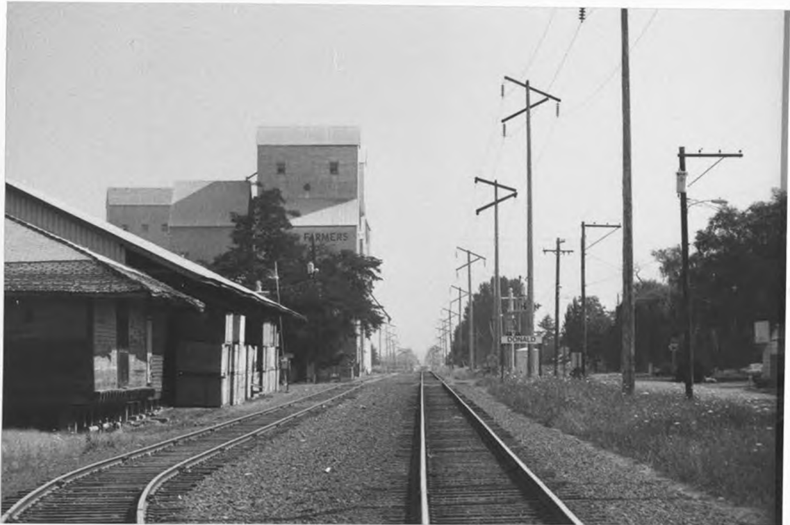
Figure 15: The rail grade divides Donald's industrial strip from a middle-class residential district.
