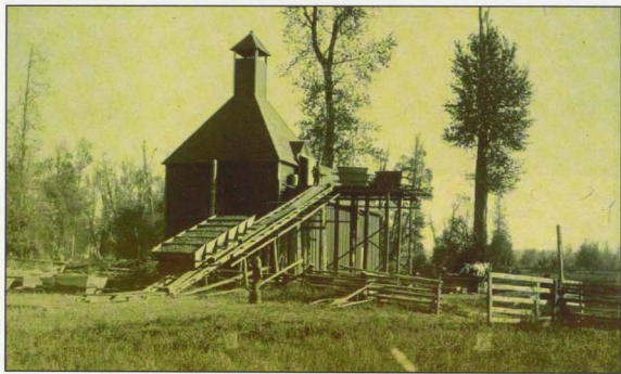
Fig. 1.3 Circa 1889 hop drier in rural Washington, demonstrating plentiful access to timber and usage of ramp and elevator systems to aid in loading. Image courtesy of University of Washington Digital Collections.
