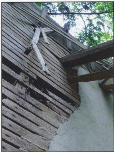
Fig. 3.3 For insulation purposes, lath and plaster covered the interior of the drying room from the ground to the bottom of the plate. Photograph by author.
