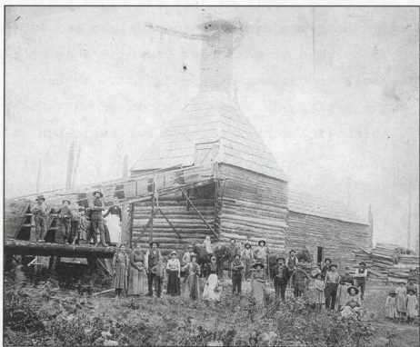
Fig. 1.2 A large and productive Washington hop drier, circa 1893. Note the vernacular construction using notched log construction for the main drier room. Image courtesy of Washington State Libraries Digital Collections.
