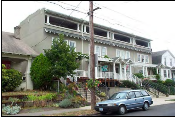
Four-level rowhouses whose height is broken up by porches, recessed balconies, and by partially excavated parking.
