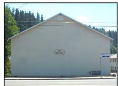
Apartment building on a commercially-zoned main street. Meets transit street setbacks and front parking limits, which are intended to foster transit- and pedestrian-oriented design, but the lack of windows works against this intent.
