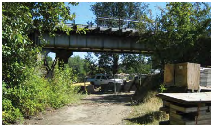
Railroad bridge and access road at north end of site
