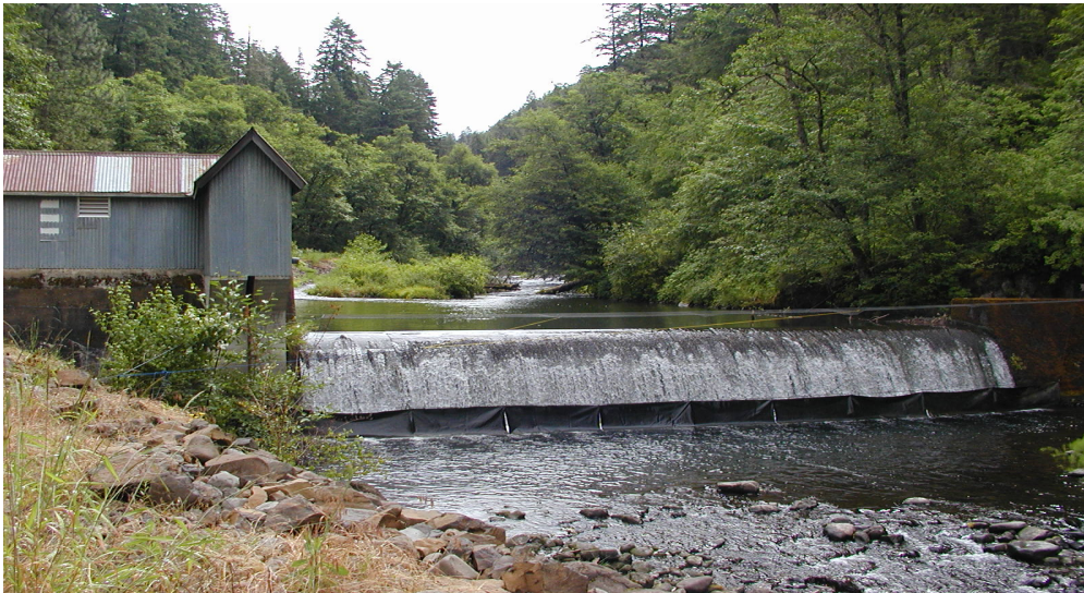
Municipal Watershed Intake Facility
