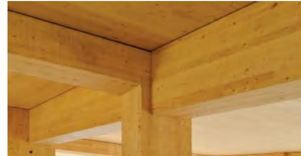
FIGURE 57 | Post and Beam Structure. (Leers Weinzapfel Associates, 2017)
