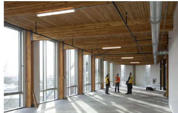
FIGURE 81 | Bullitt Center in Construction. (Bullitt Center Staff, 2013)
