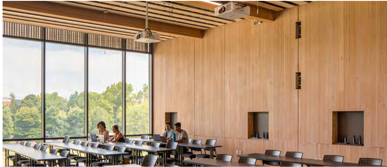
FIGURE 41 | Interior View of CLT Rocking Shear Walls (Josh Partee, 2020)
