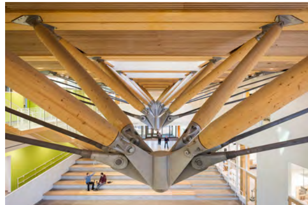
FIGURE 61 | Zipper Truss System. (Leers Weinzapfel Associates, 2015)
