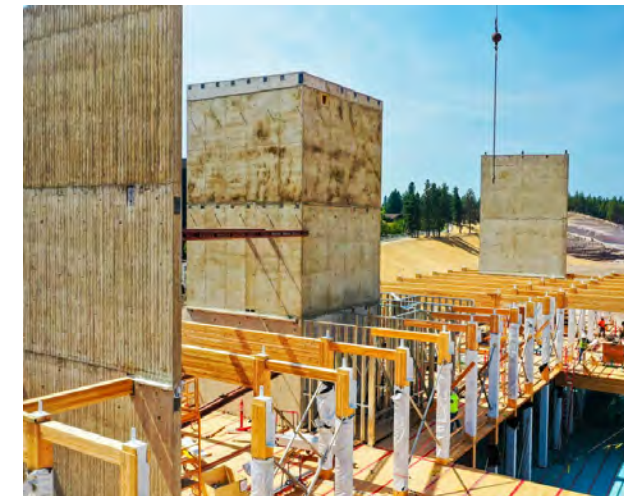
FIGURE 101 | Concrete Shear Walls in OSU Cascades. (SRG Partnership, 2020)
