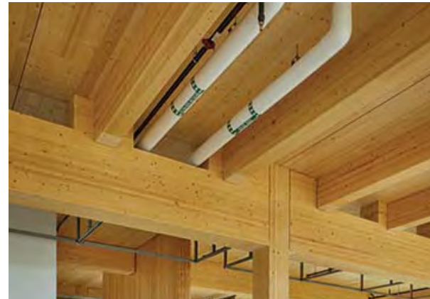
FIGURE 32 | T-Rib CLT Floor Panels (Michael Green Architecture, 2021)
