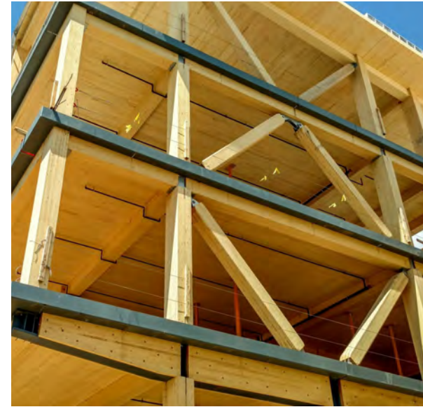
FIGURE 62 | Lateral Bracing System. (Woodworks, 2018)
