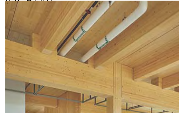
FIGURE 3 | Timber T-Rib Composite Panels. Catalyst in Spokane, WA. (Benjamin Benschneider, 2020.)
