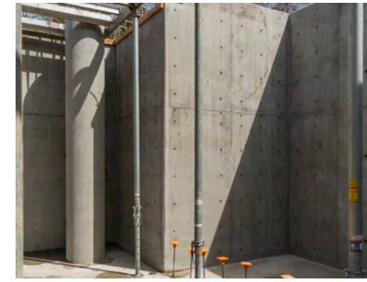
FIGURE 110 | Tykeson Hall Concrete Column and Walls. (Josh Partee, 2018)
