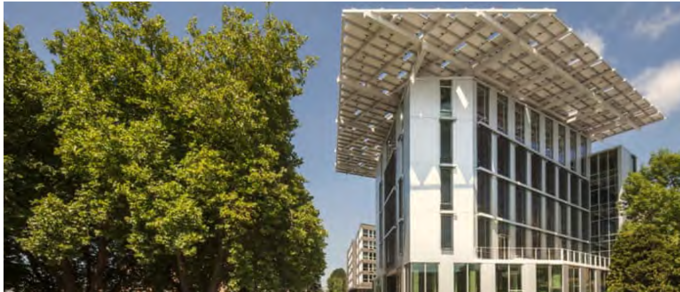
FIGURE 78 | Exterior View of the Bullitt Center in Seattle WA. (DCI Engineers, 2013)
