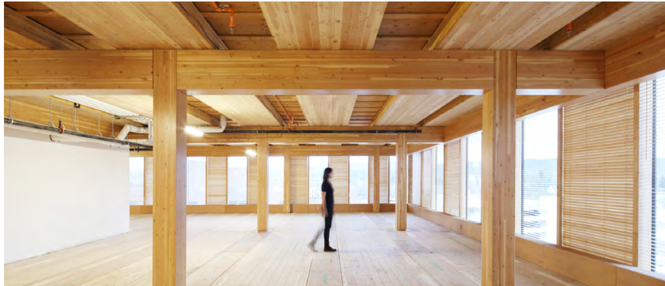
FIGURE 50 | Interior View of Mass Timber Structure. (Michael Green Architecture, 2015)
