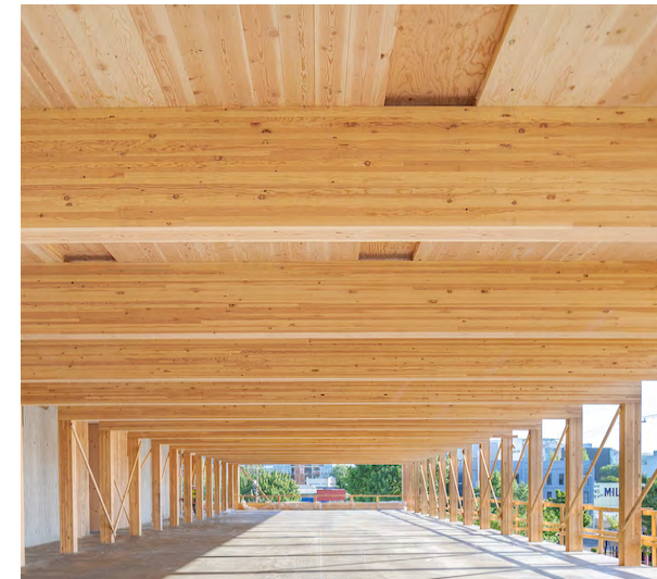
FIGURE 9 | Mass Timber Structure at District Office, Portland OR. (Structure Magazine, 2020)
