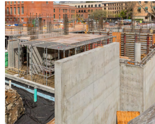
FIGURE 109 | Tykeson Hall Concrete Structure in Construction. (Josh Partee, 2018)
