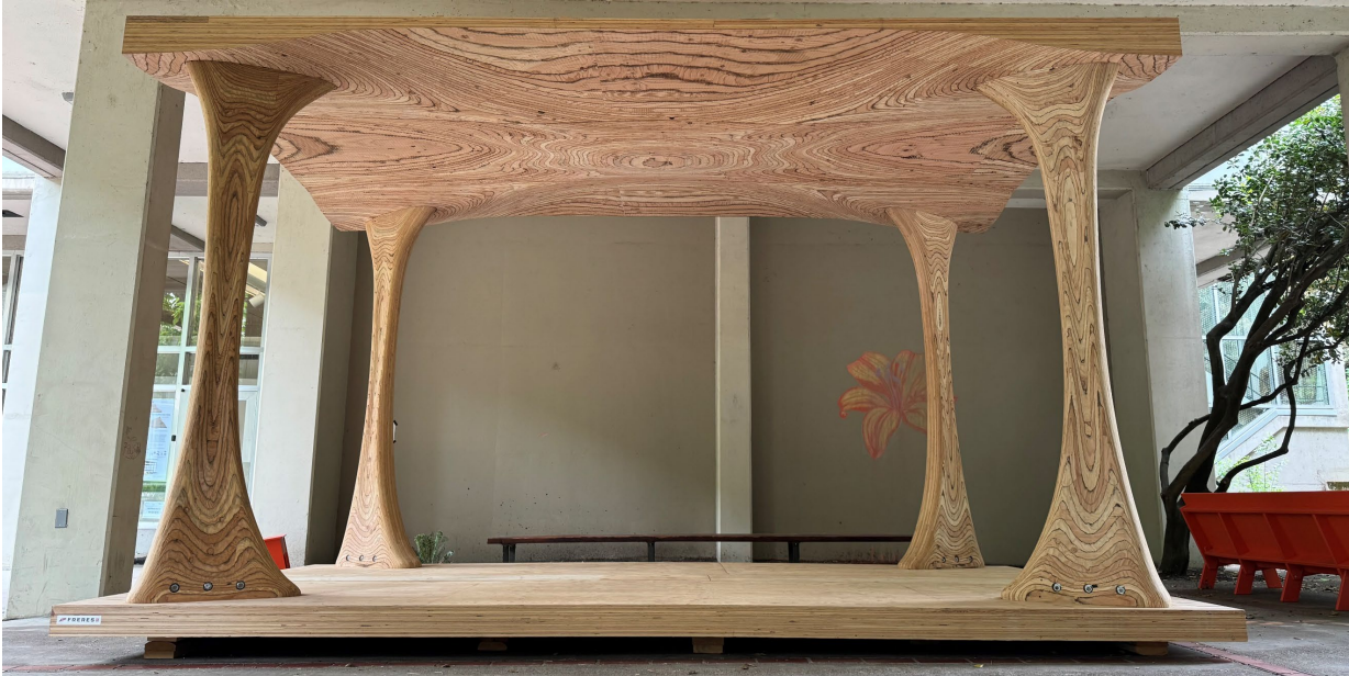
Figure 8. Pavilion exhibition completed for the 2024 International Mass Timber Conference
